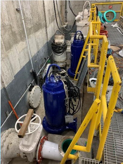
Installation of two new pumps
