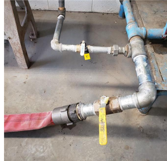
In March, the Meter department made improvements to the meter test bench; reducing test times from an hour to 15 minutes. Dustin Mills and Derrick McMichael came up with an idea to fix the current water tank drainage problem. They cut the pipe and installed a ball valve; making it possible to drain the water more quickly through a hose. They also mounted a shelf for added organization. These improvements will help the meter department test  $\frac{3}{4}$ " to 2" meters more efficiently.
