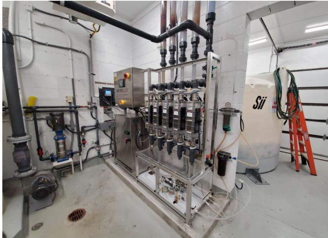
Fig 1.: Example Chlorinator at Well No. 8
