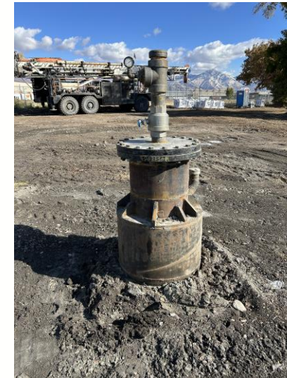
Well Capped Off
