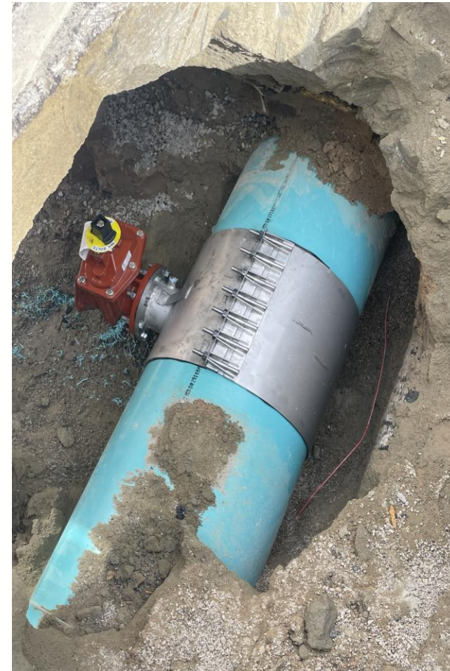
8" fire line and PVC coupon from hot tapping process
