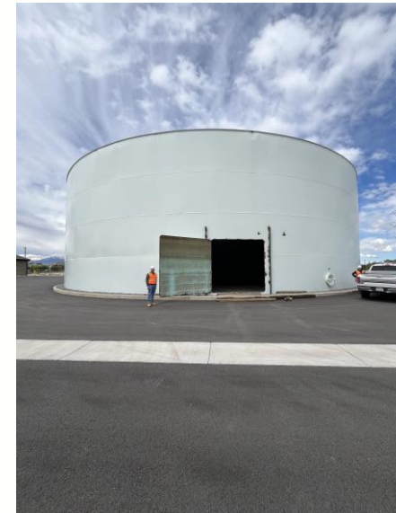
Acord Reservoir Tank
