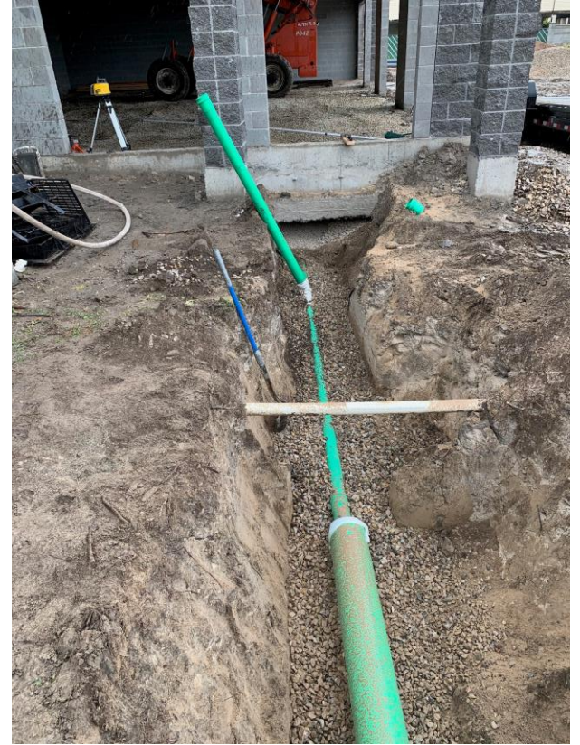
Sewer cleanout near building
