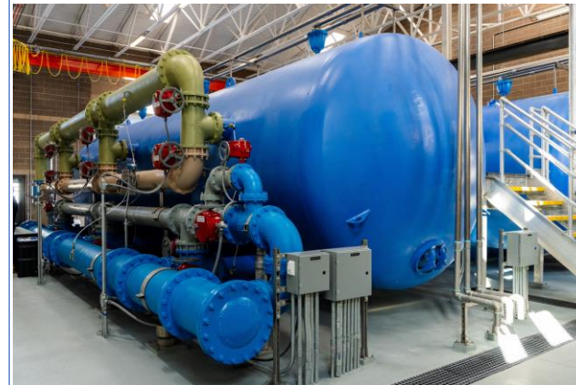
Completed Filter Vessel
