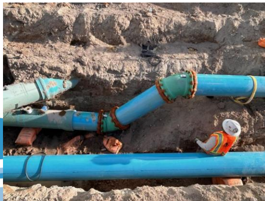
Installing 16" PVC waterlines
