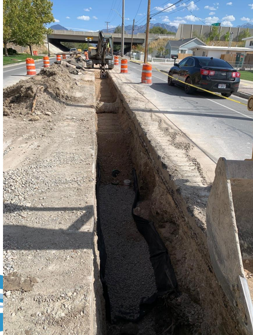
10" sewer main trench
