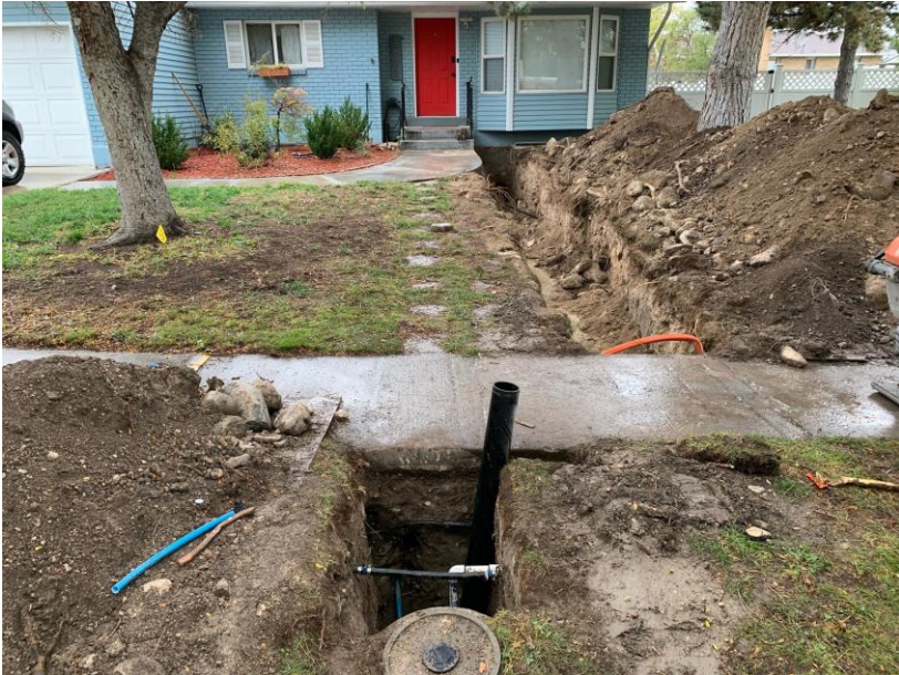
Water lateral trench in park strip and yard
