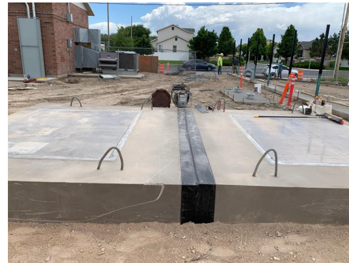
Mastic Seal Tape on Interceptor Vault
