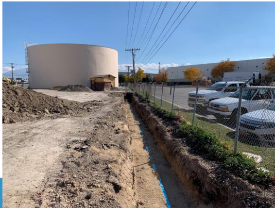
16" WTR line trench
