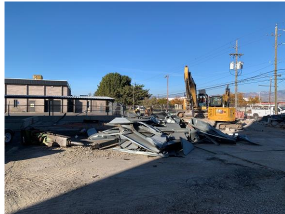
Pumphouse and generator buildings demolished
