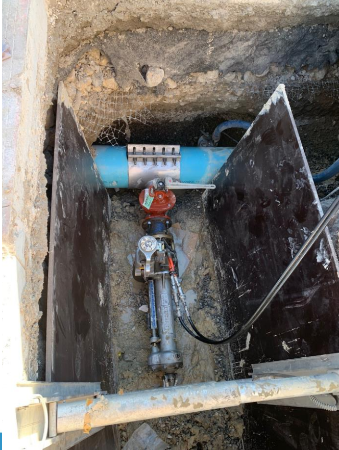
4" hot tap on 12" water main
