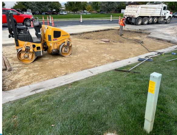
Roadway grading and compaction
