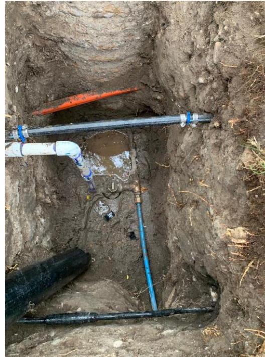
Stop and waste valve connection
