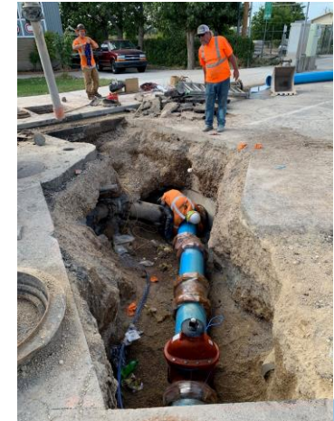
12" water main tie in
