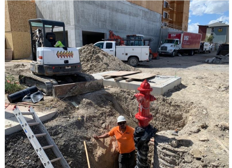
Hydrant installed on 8" fire line stub in
