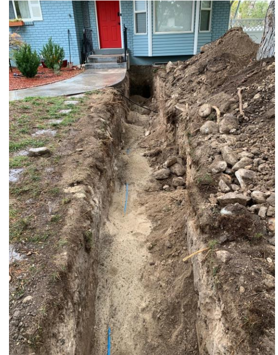
Water lateral bedded in sand
