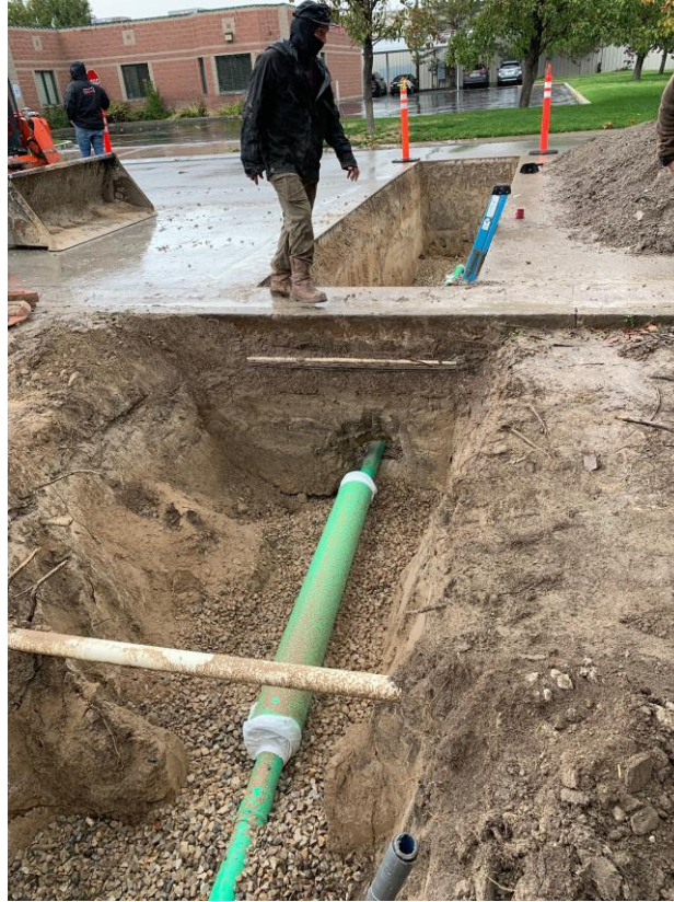
4" sewer lateral with 8" casing
