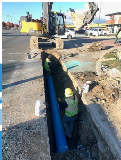
12-inch PVC Installation
