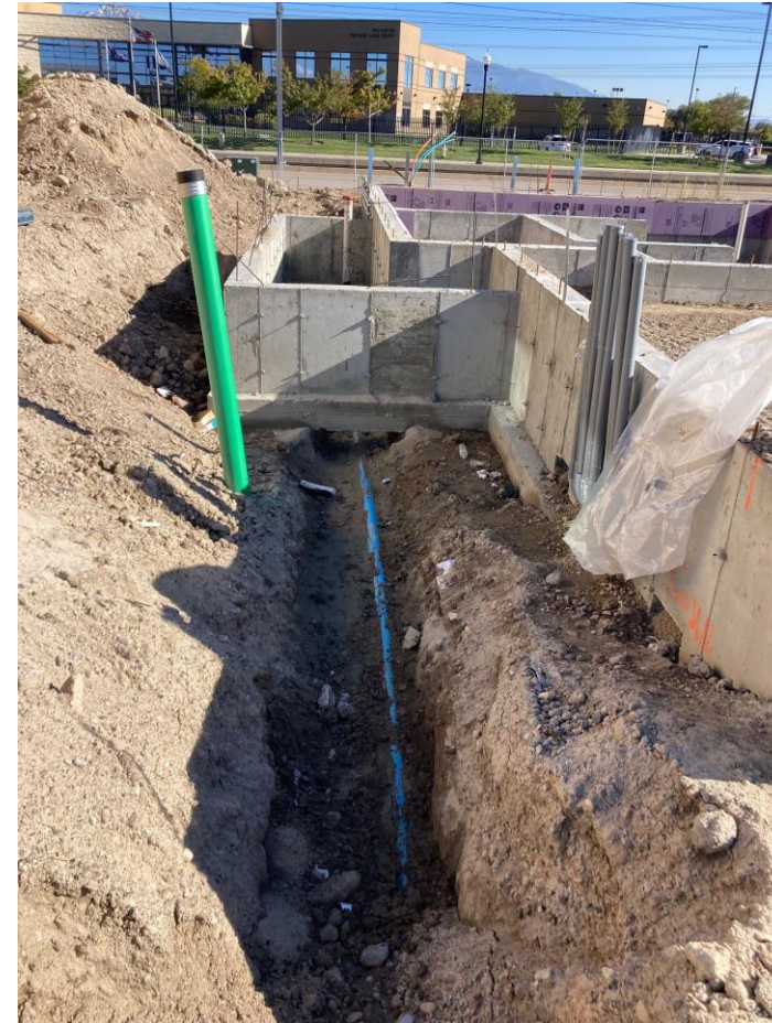
4" fire line with sand bedding and tracer wire
