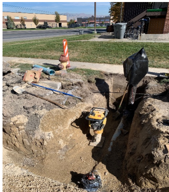
Fire Hydrant backfill
