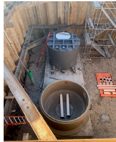
Wet well and dry well progress
