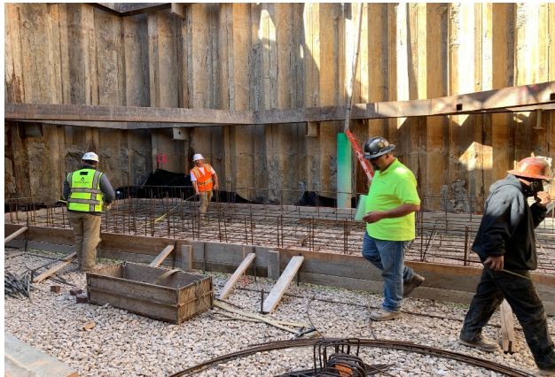
Formwork for wet and dry well pad
