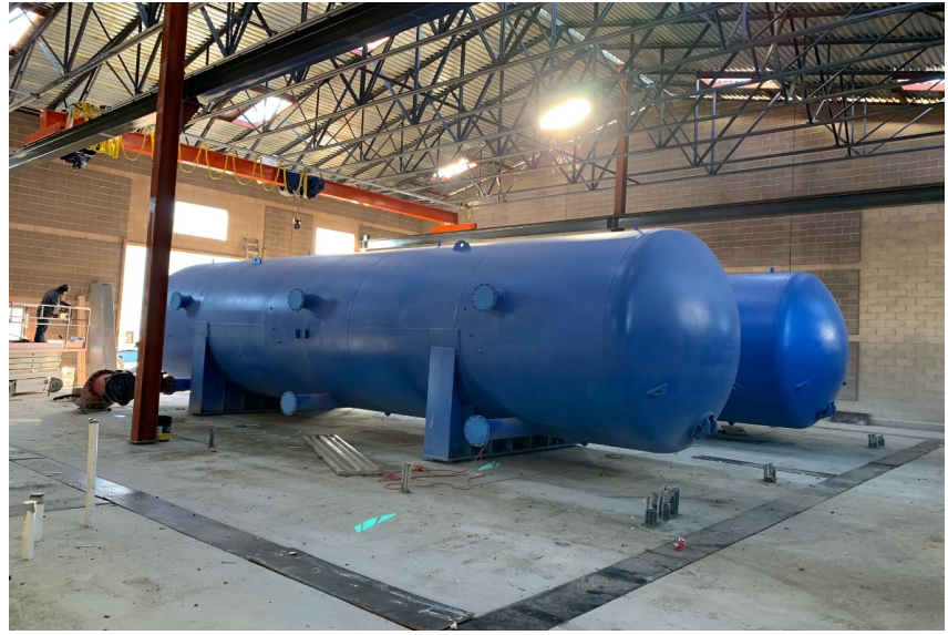
Roof and crane installation
