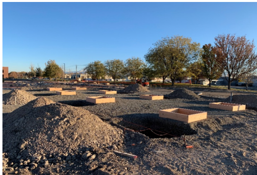
Pavilion foundations and forms
