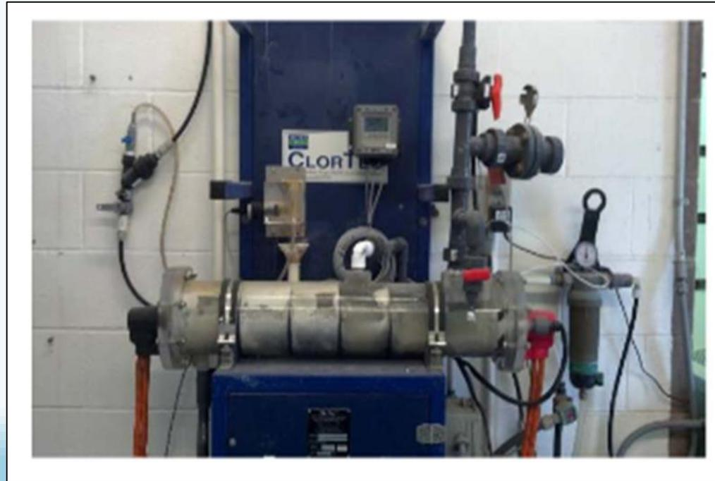
The picture above is the old sodium hypochlorite generation system that was replaced with the new PSI system at Well 8 in 2020.
