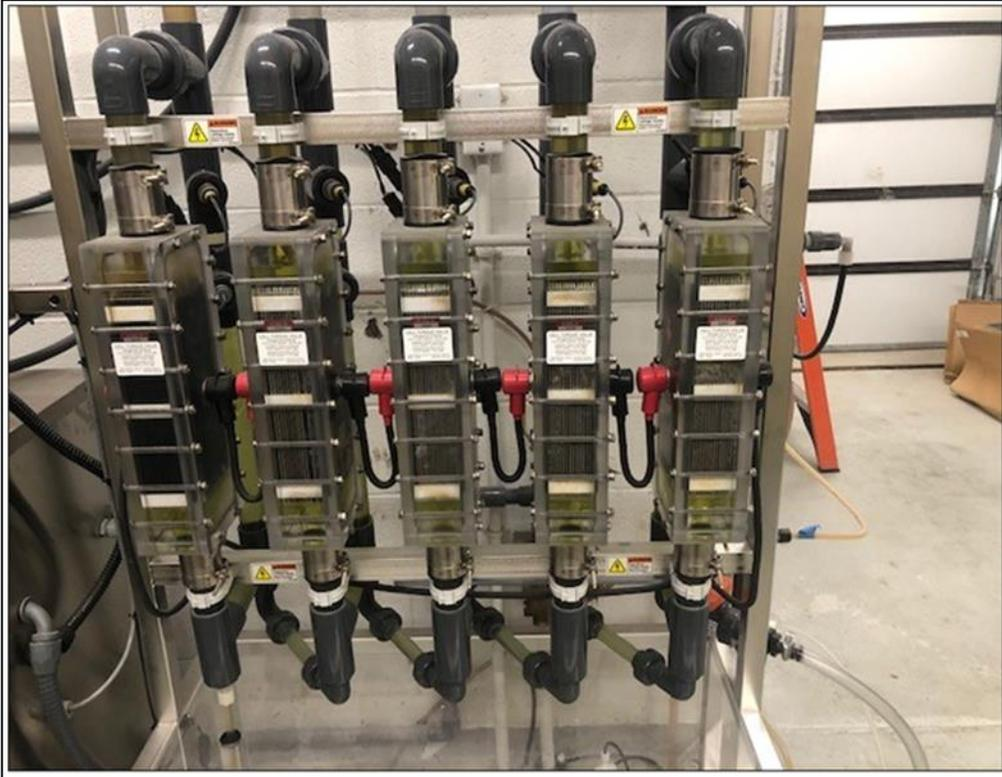
The picture to the left shows the sodium hypochlorite cells at Well 8 during the cleaning process. They are being cleaned with a hydrochloric acid solution mixed at a 1:4 ratio of acid and water. The cells are first drained, and the solution is then pumped into the cells. The acid solution remains in the cells for 15 to 20 minutes, giving the solution the necessary contact time to clean and dissolve any buildup of sodium in the cells that can cause the system to run poorly.
