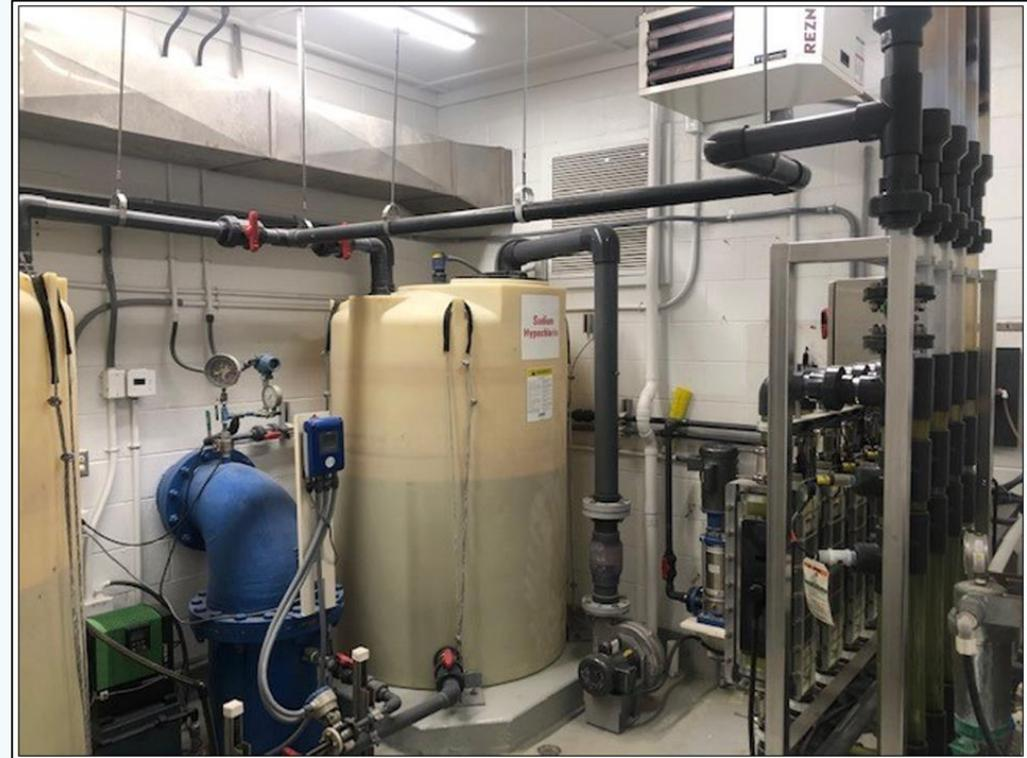
The picture above is the inside view of the sodium hypochlorite room at Well 8. The large tanks to the left of the picture are the storage tanks for the sodium hypochlorite solution that we use to disinfect our water. To the right of the picture is a side view of the new PSI sodium hypochlorite generation system. The new system was installed and put into operation in July of 2020.
