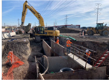
Trench shoring and dewatering setup
