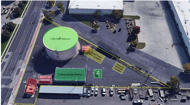
Ridgeland Pump Station and Reservoir Site
