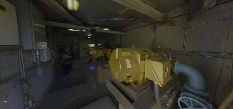
Interior of existing pump station
