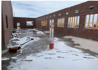
Building Addition - Completion of masonry work for the addition
