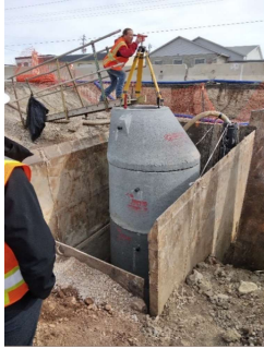
First manhole for incoming gravity line
