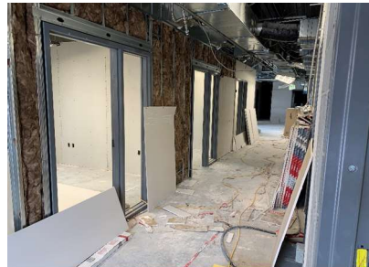
Building Remodel - Framing and insulation for main
