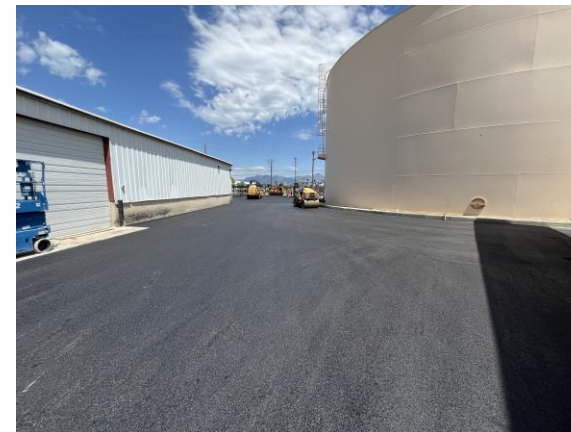
Asphalt Site Paving
