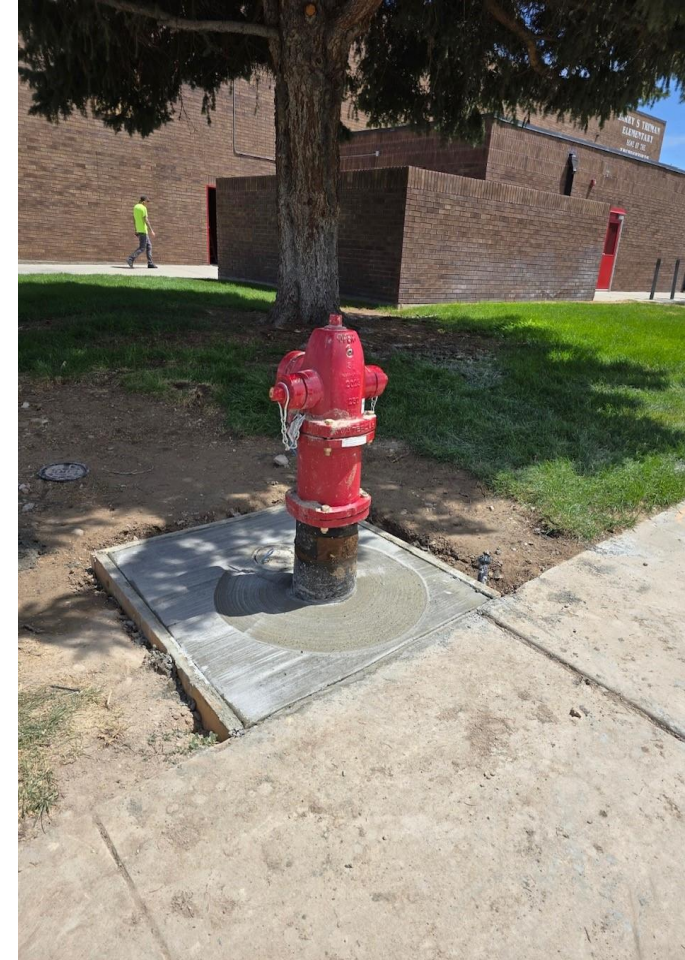
New fire hydrant install
