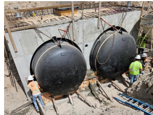
Surge tank vault
