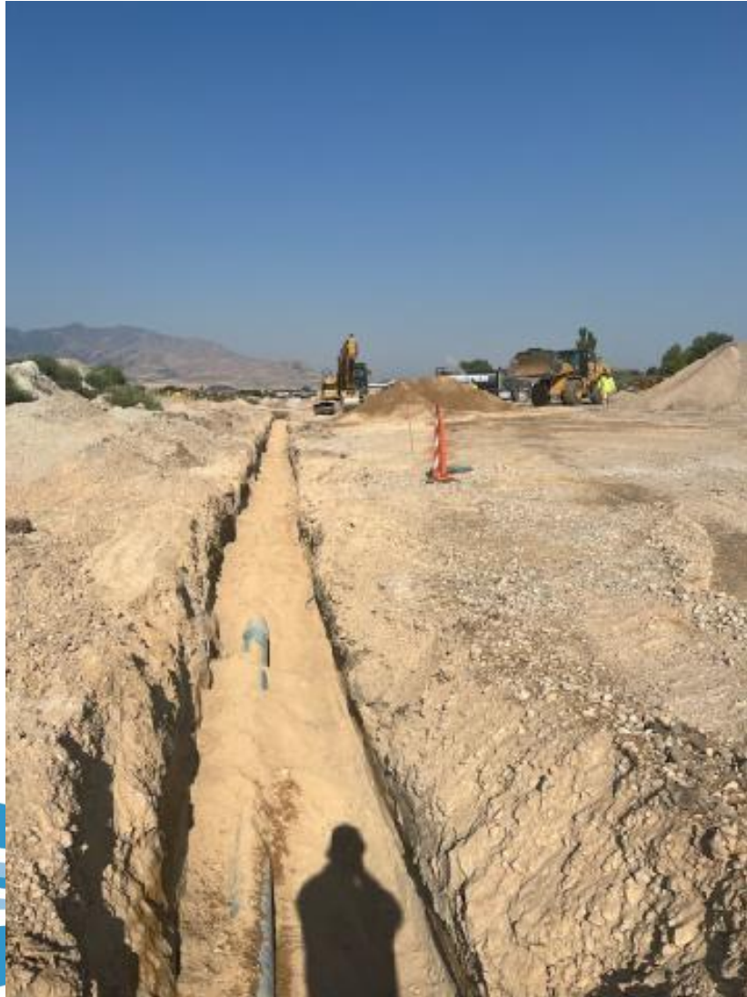
8" water main trench with sand bedding
