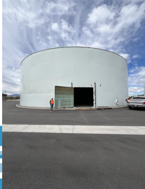
Acord Reservoir Tank
