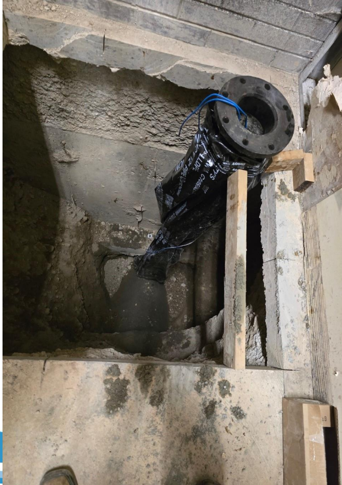
6" fire riser upgrade
