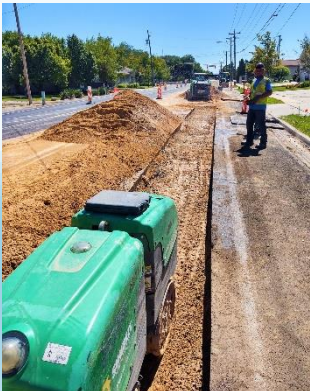
Trench compaction with remote-controlled compactor
