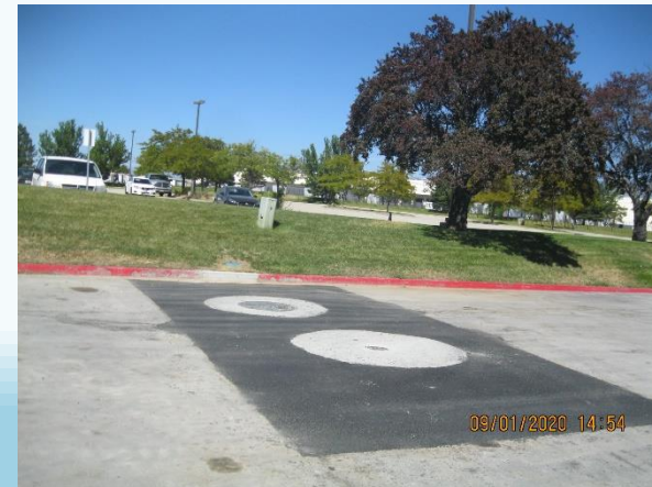
Final surface restoration at Franklin Covey south meter vault
