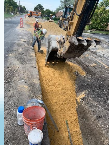
Trench backfill and compaction
