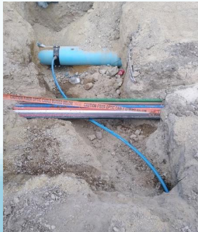
New water service lateral at 5427 West installed under existing fiber lines.
