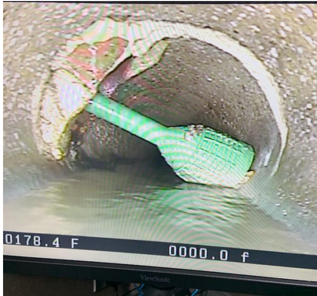
Figure 9: Depicts a snowball maker/thrower coming out of a lateral into our sewer main on 2200 W.
