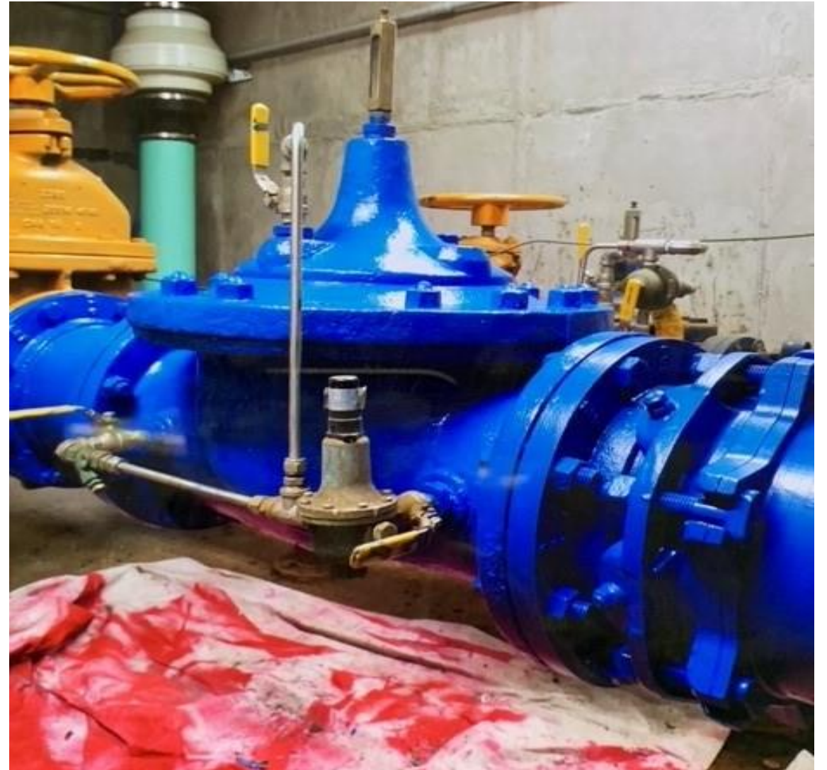
PRV after repairs / maintenance completed and new coating system applied.
