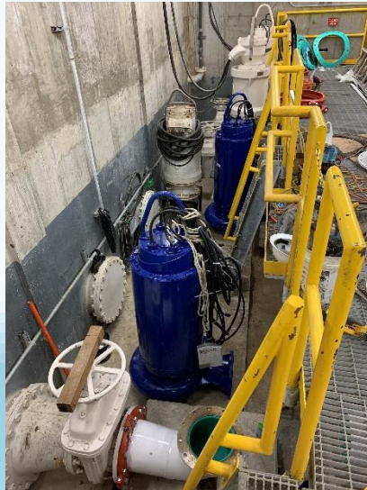
Installation of two new pumps
