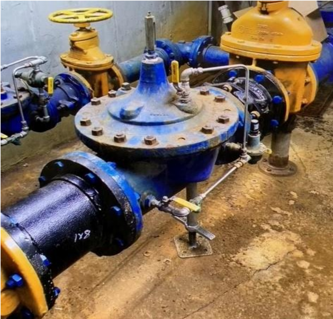
PRV after repairs / maintenance and prior to coating application.
