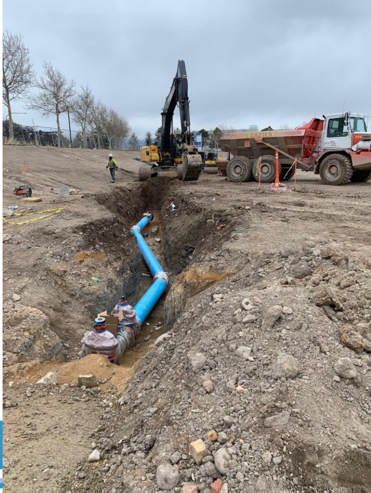
New waterline with fittings and valves
