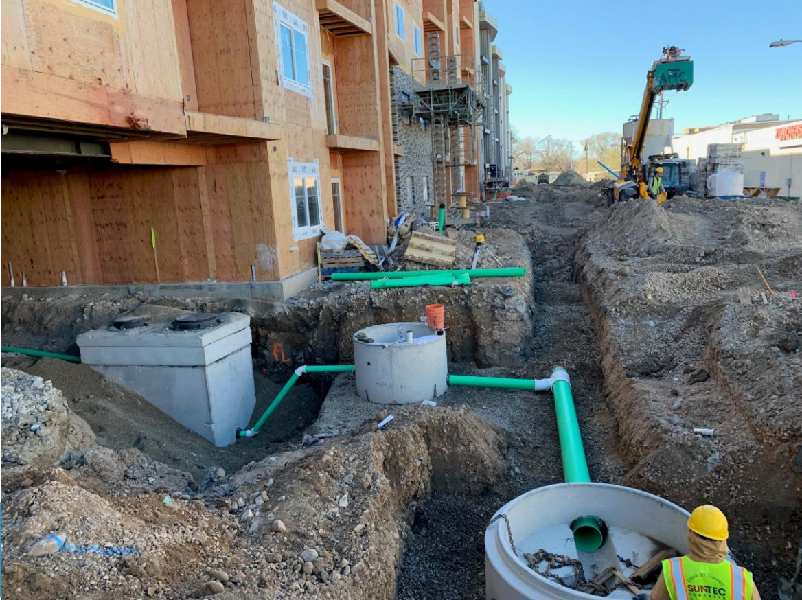
Installed grease interceptor, sampling manhole and sewer main/manhole
