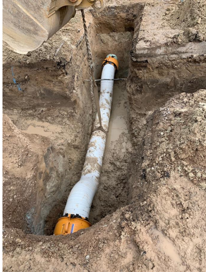
12" prefabricated steel waterline loop
