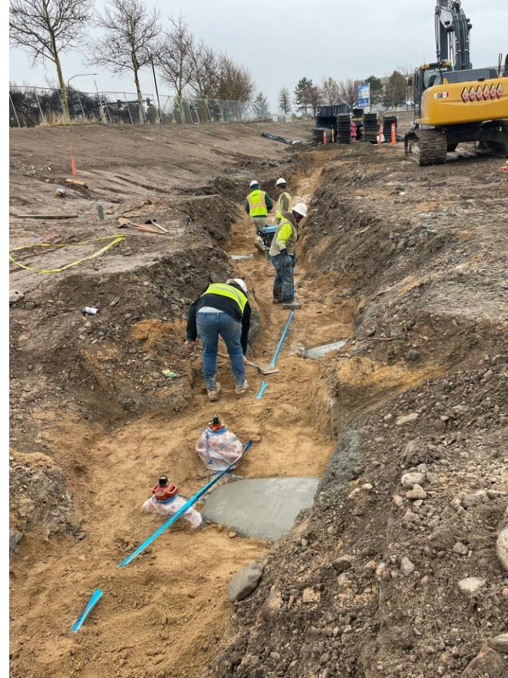
Pipeline and fittings with thrust blocking and backfill material
