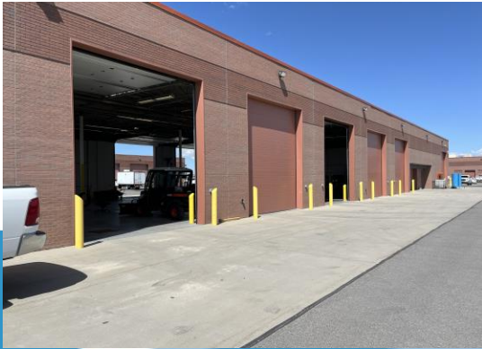
Newly installed garage doors in operation
