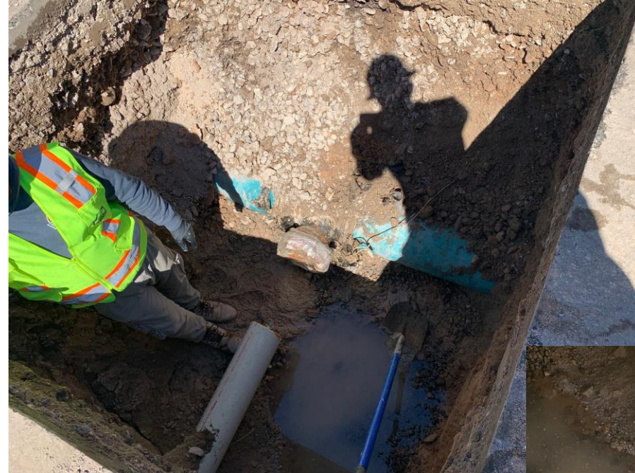
Abandoned 6" water main with a plug at the end
