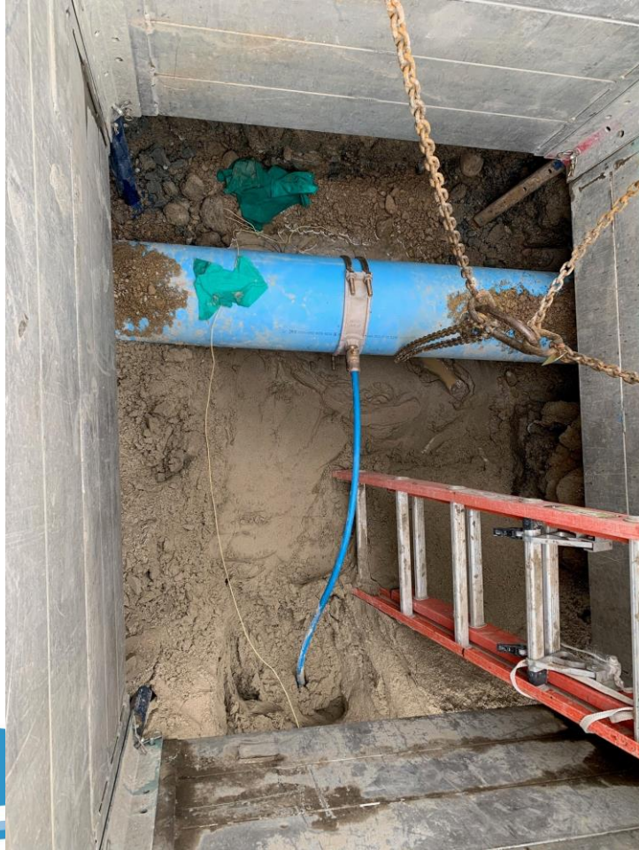
3/4" brass saddle tapped on 12" water main
