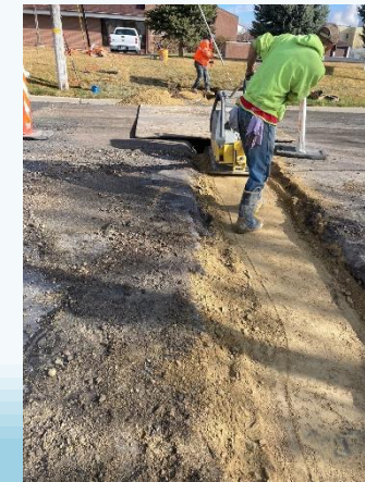
Laborer compacting trench for water service line
