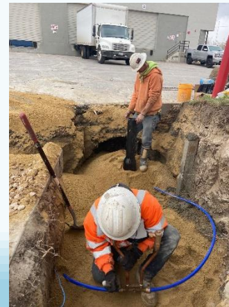
Meter assembly installation at 2215 W. 2200 S.
