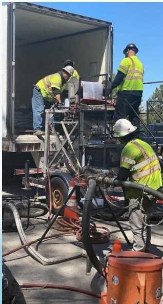
15-inch CIPP installation
