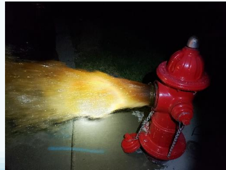
Flushing in progress
