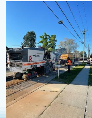
Milling machine at work on 2200 West
