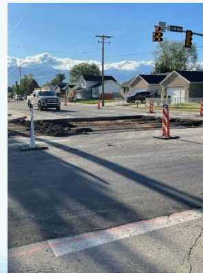
Preparing to pave the 3800 S. 2200 W. intersection
