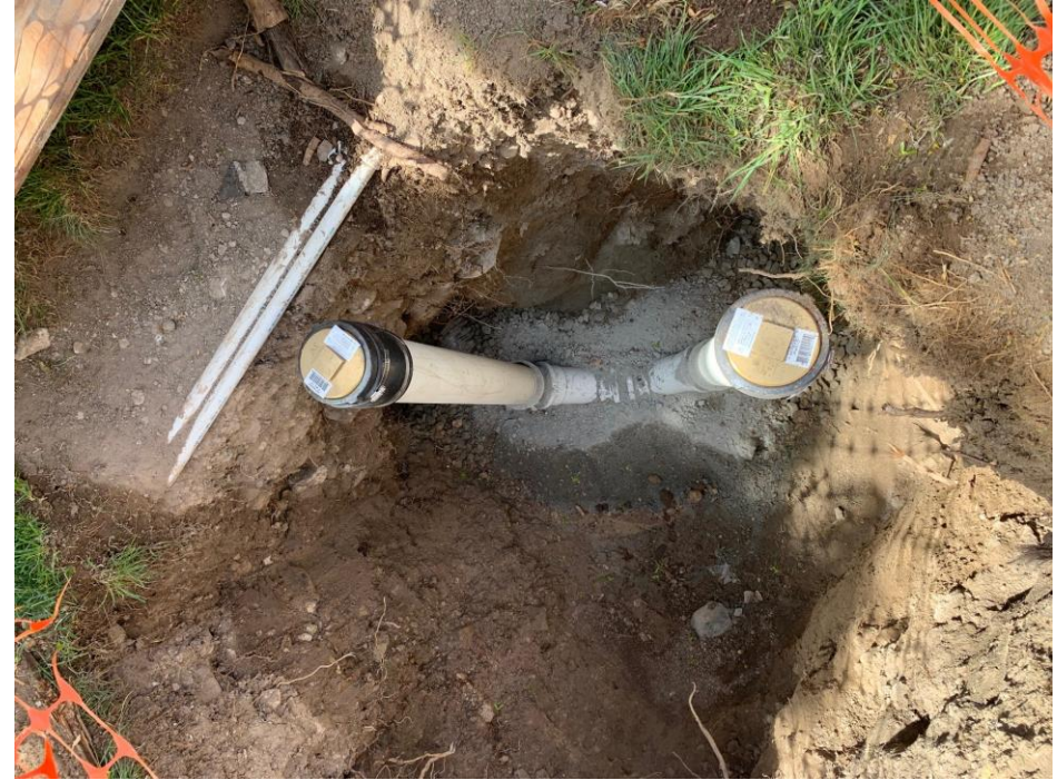
Cleanouts with gravel bedding
