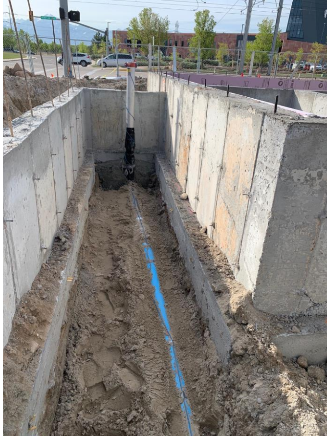
4" fire riser inside building
