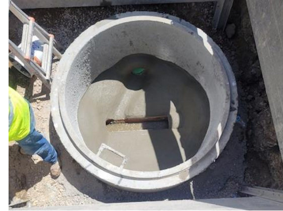
Finished cast-in-place manhole base
