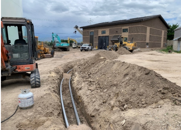
2-inch conduits running toward treatment facility
