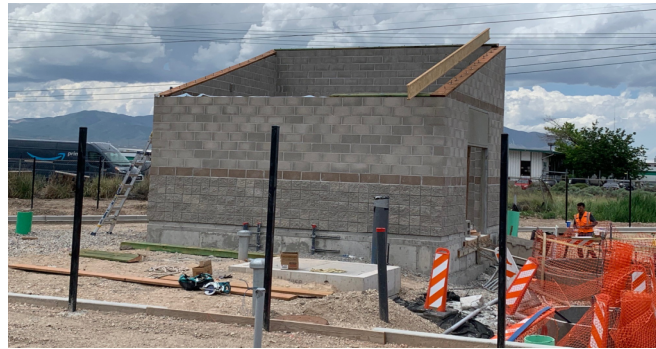
Pump station building with roof trusses being installed
