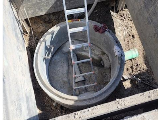
Working on manhole bench and trough
