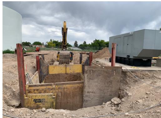
Shoring for chlorine vault
