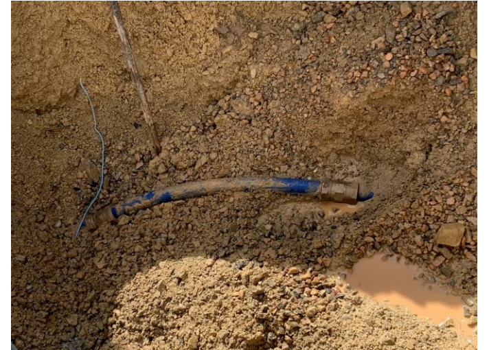
Water lateral repair with compression fittings
