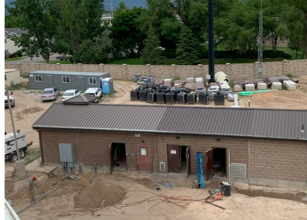
2-inch conduits running toward treatment facility
