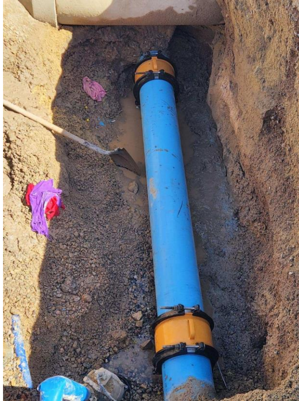
Fire line repair with Romac Alpha couplings
