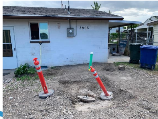
New sewer cleanouts and abandoned septic tank location
