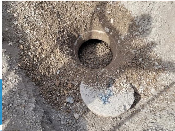
Septic tank filled with gravel prior to abandonment
