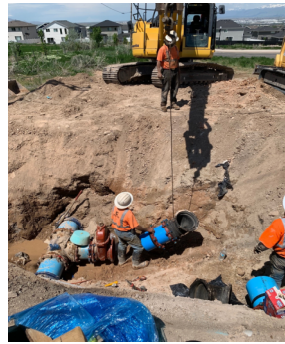
12" Connection to AC line 4700 S
