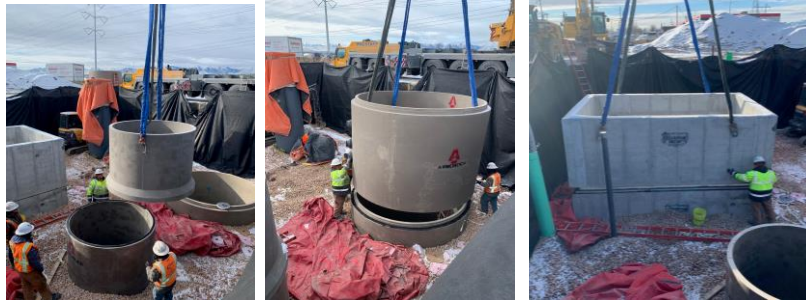
Installing sections for diversion manhole, wet well, and pig launch vault
