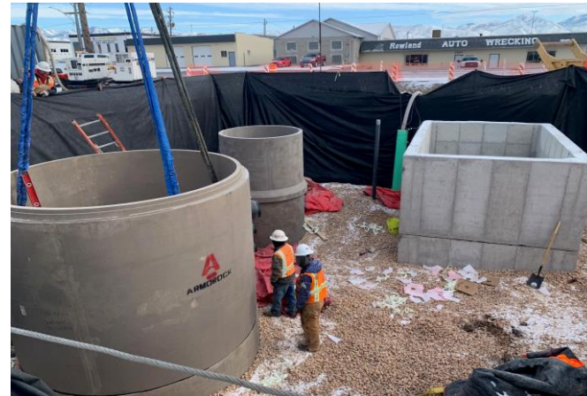
Installed wet well, diversion manhole, and pig launch vault sections
