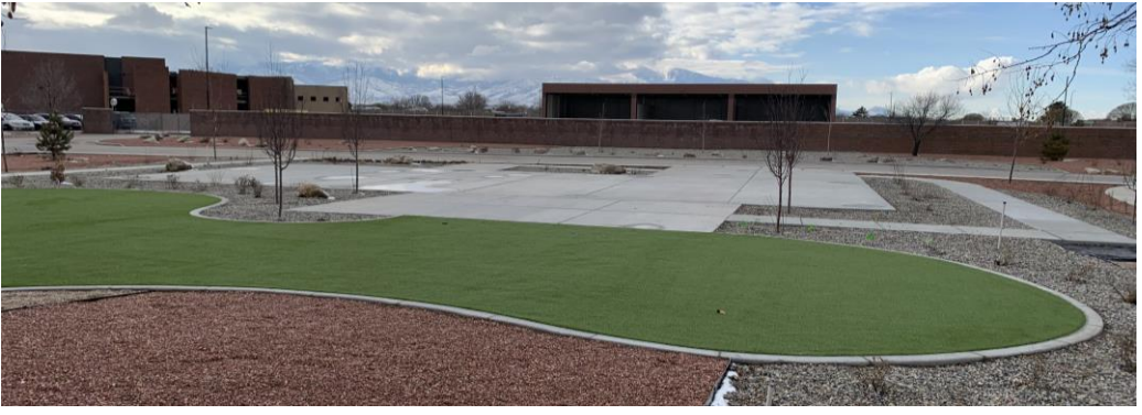
Finished concrete pad for demonstration garden area
