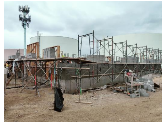
CMU installation for pump station building
