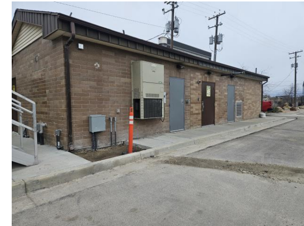
New doors and electrical work.
