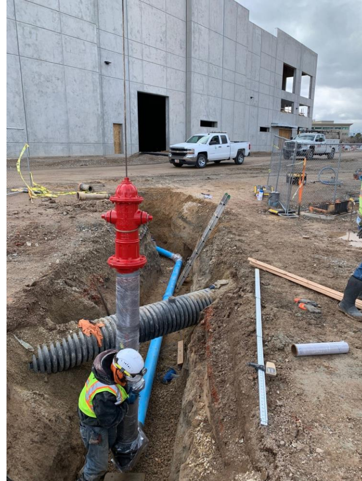
Installing a fire hydrant on the north side of the building
