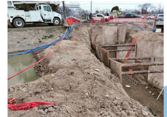
Bypass pumping of canal water around pipe installation site
