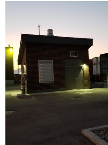
Montec Lift Station
