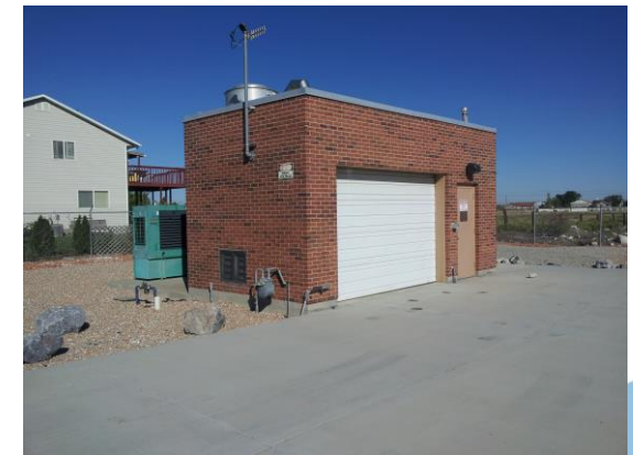
Pleasant Valley Lift Station
