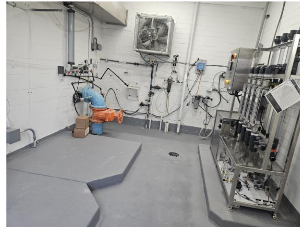
New chlorinator, epoxy flooring, and concrete pad.
