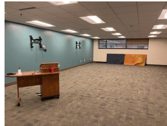
AV, lighting, and ceiling tile installation
