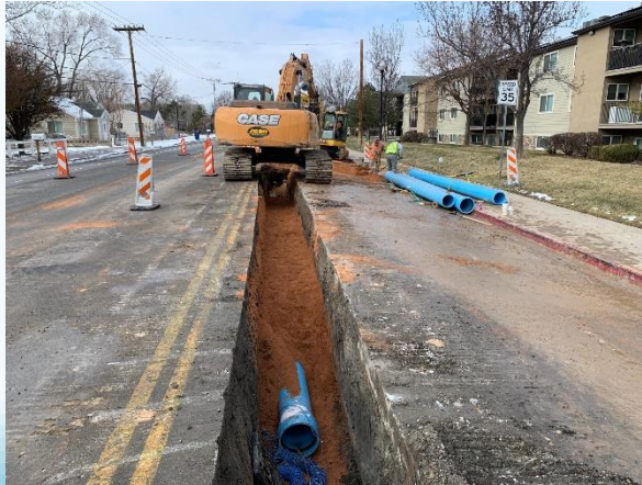
12" waterline installation west of 2200 W. 3800 S. intersection
