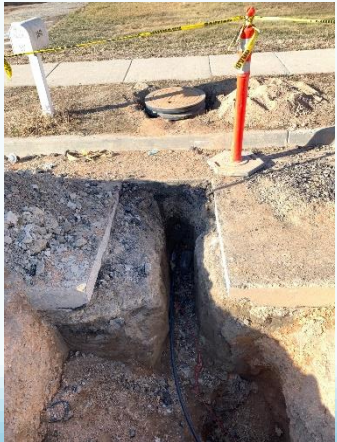
Meter box and trench for water service at 3850 S. 2200 W.
