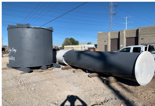
Dry well and access tube
