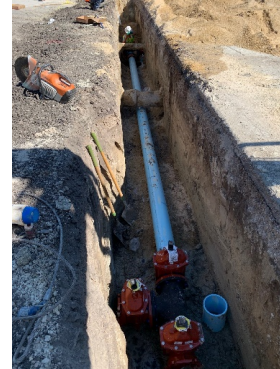
Fusible PVC installation
