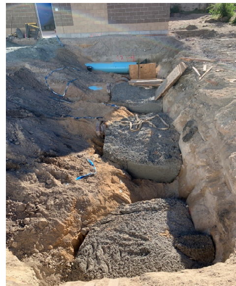
Thrust Blocks for 24-inch waterline
