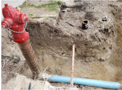
Fire Hydrant Installation
