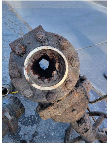
Build-up around pipe
