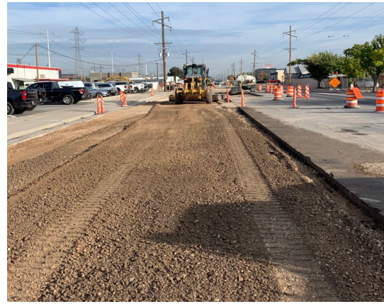
Grading in preparation for asphalt placement on Constitution Blvd.
