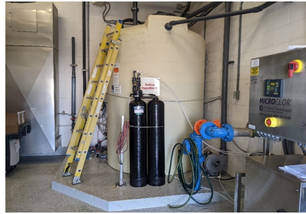
Well No. 15 Soft water tank and blower installation
