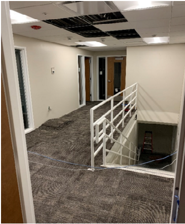
Carpet Installation in Mezzanine
