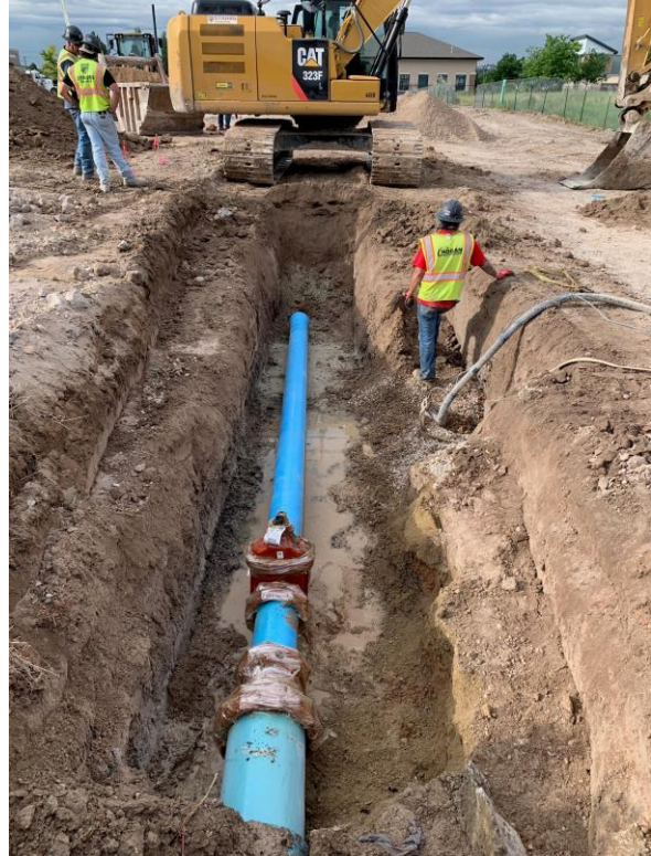
Waterline tie in with 12"x8" reducer and 8" gate valve
