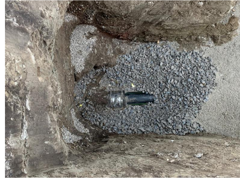
Connection at sewer main
