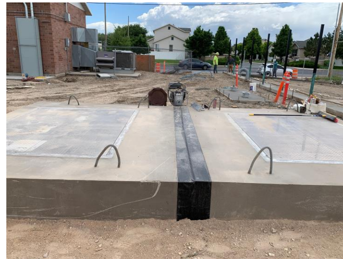
Mastic Seal Tape on Interceptor Vault
