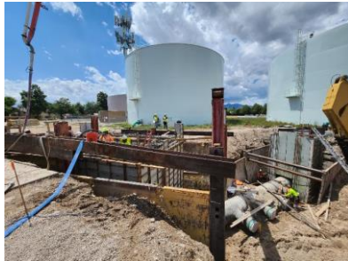
Concrete truck pumping concrete for chlorine injection vault walls
