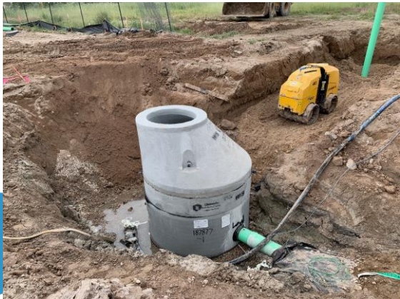
Manhole connection
