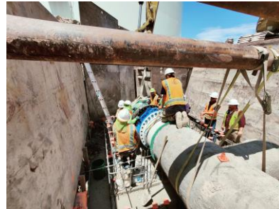
36" double eccentric butterfly valve vault - piping and valve installation
