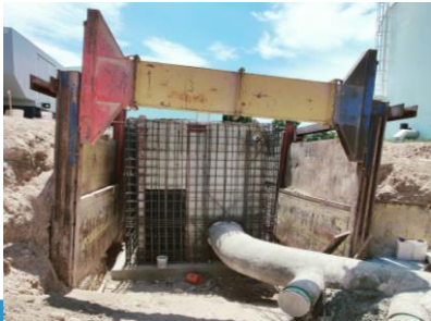
Chlorine injection vault rebar - north end
