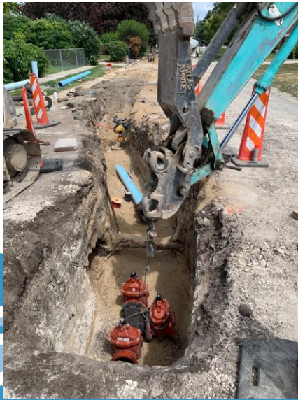
Tee installation along Merry Ln & Sunshine Dr
