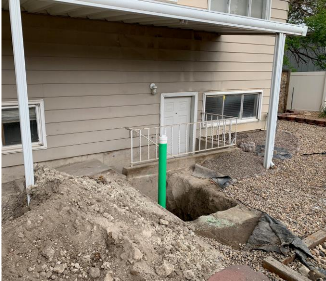
Cleanout location near property
