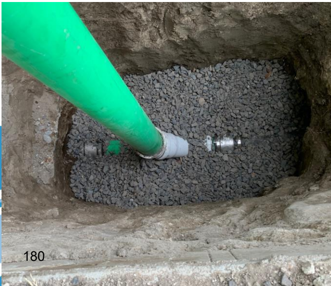
Gravel bedding in cleanout trench
