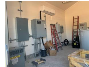
Panels on east wall of building
