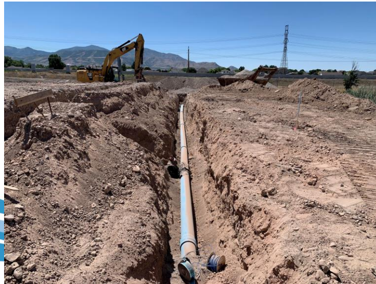
8" waterline installed on north side of building
