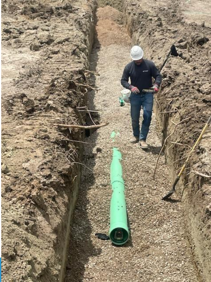
8" sewer with grade laser inside pipe
