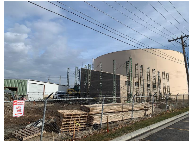
Booster pump station CMU wall installation
