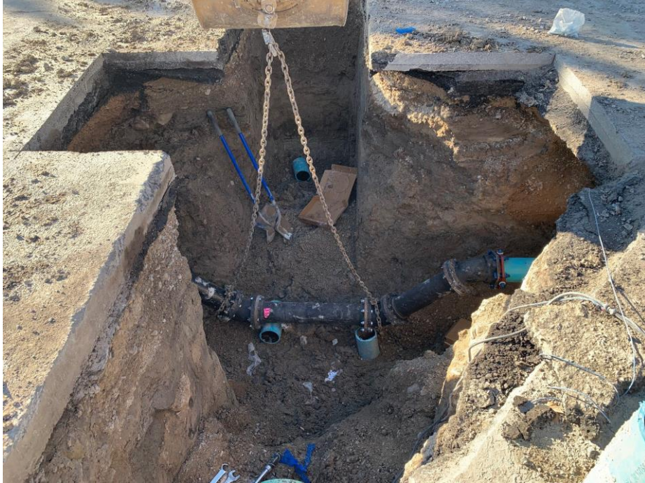
6" ductile iron waterline loop
