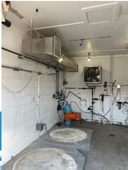
Demolition of tanks
