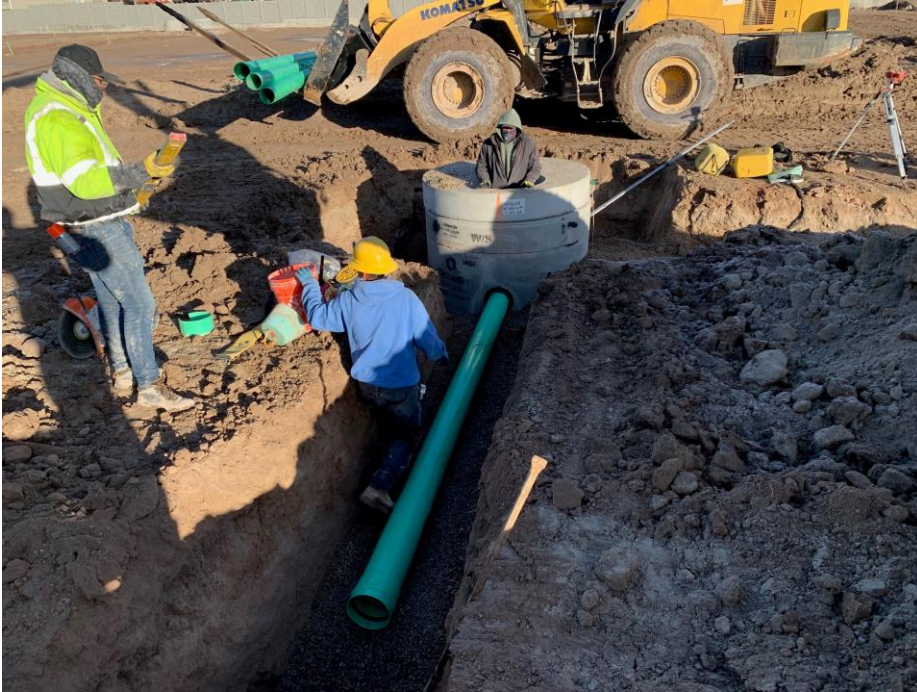
Installing pipe in manhole
