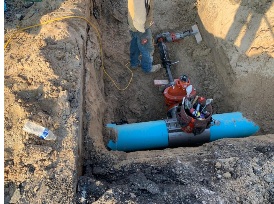
8" hot tap on 12" water main
