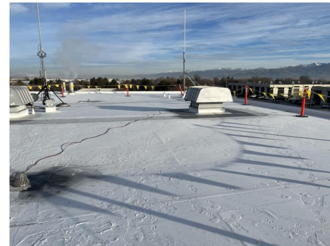
Newly installed membrane
