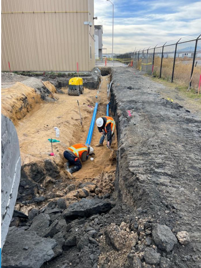
Installing sand bedding for 4" and 6" waterlines
