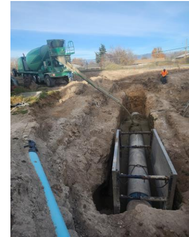
Backfilling pipe with flowable fill
