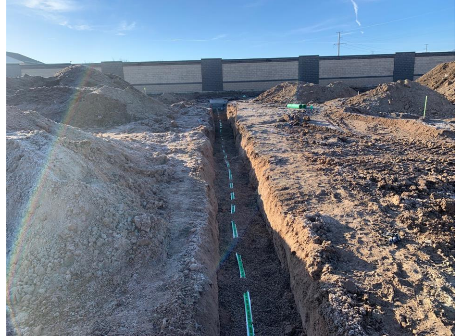
Sewer trench with gravel backfill and warning tape
