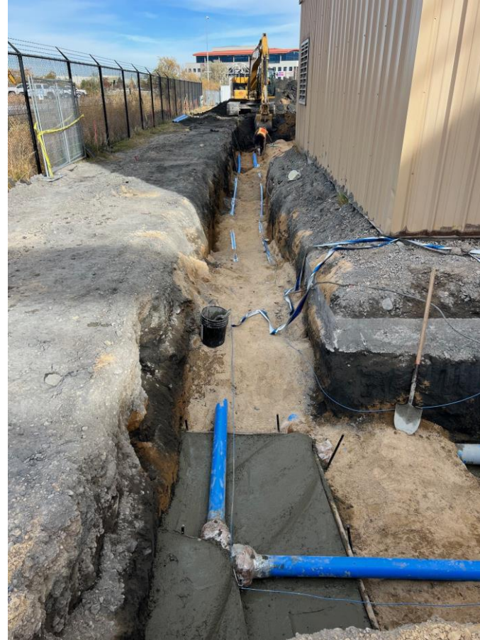
North view of trench with thrust block on 4" waterline fitting
