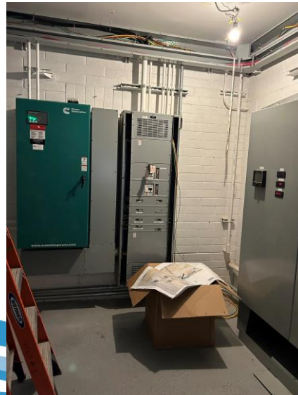
Installation of electrical work
