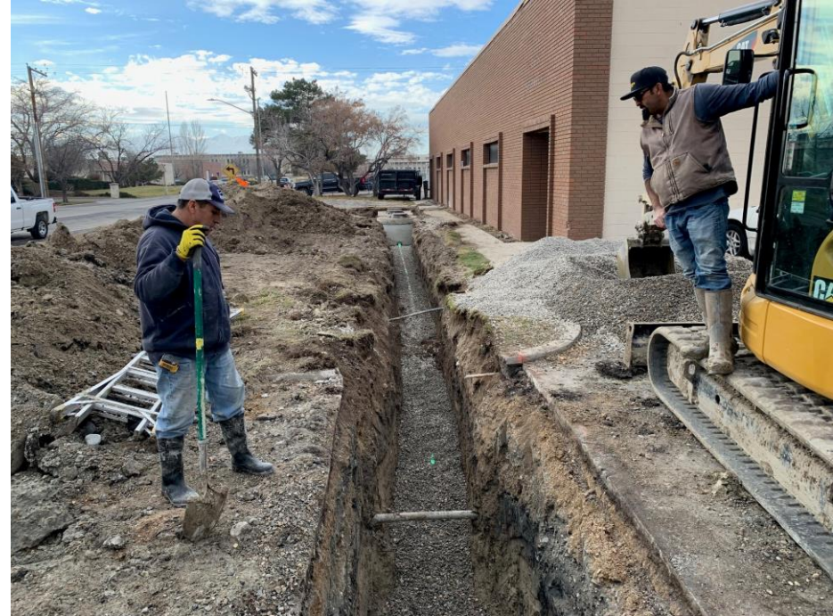
View of grease line sewer trench
