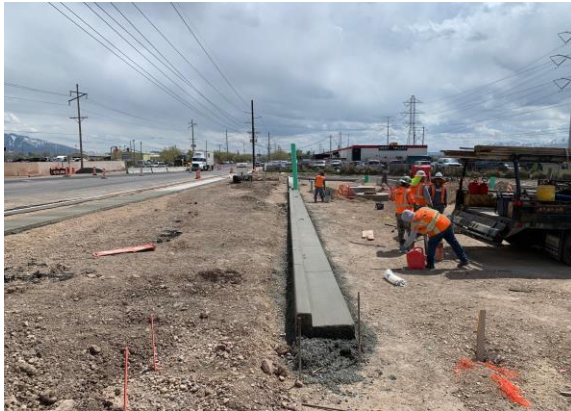
Sidewalk and curb and gutter installation
