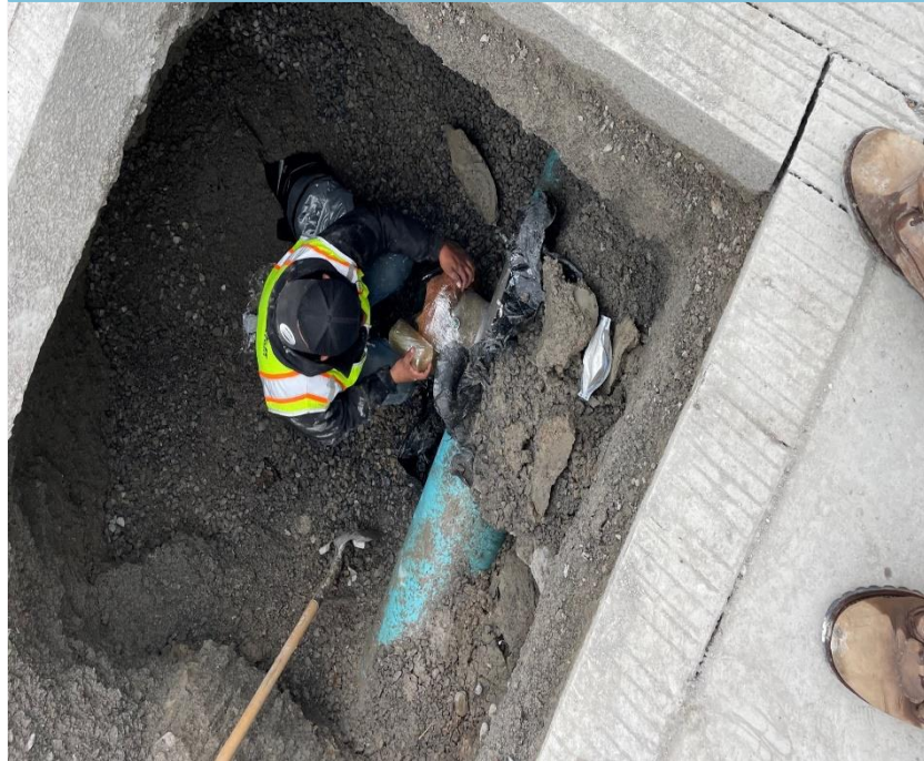
Post valve removal - wrapping capped tee and pipe with wax tape and poly-ply wrap
