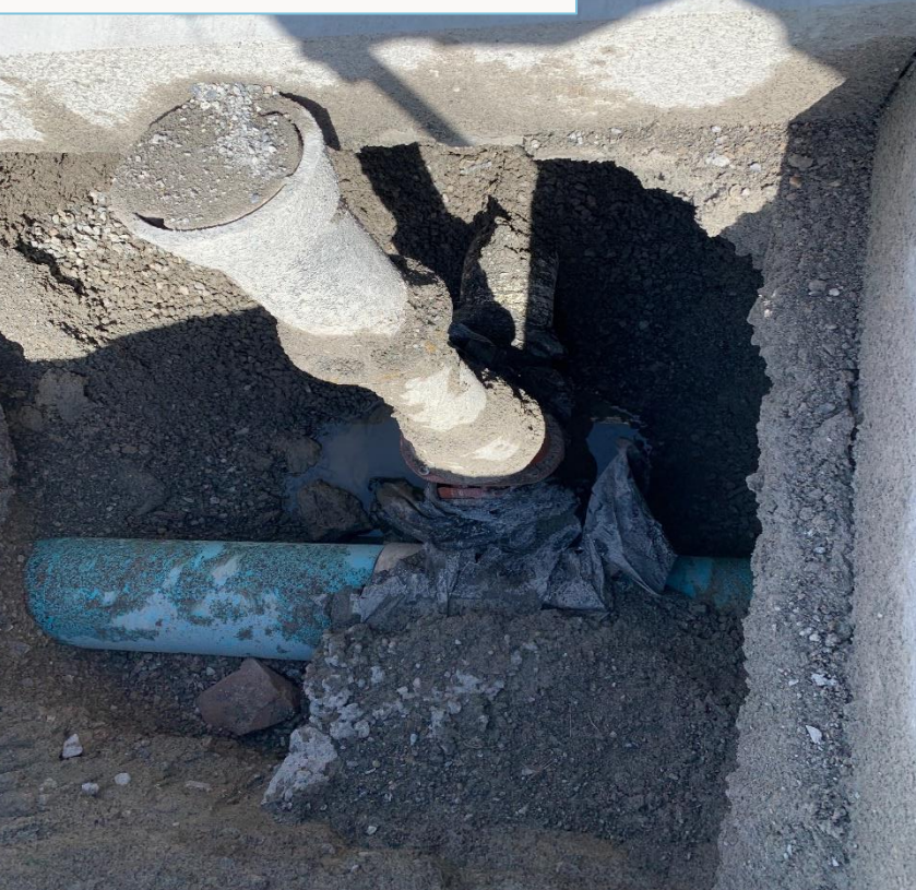
8" valve prior to removal
