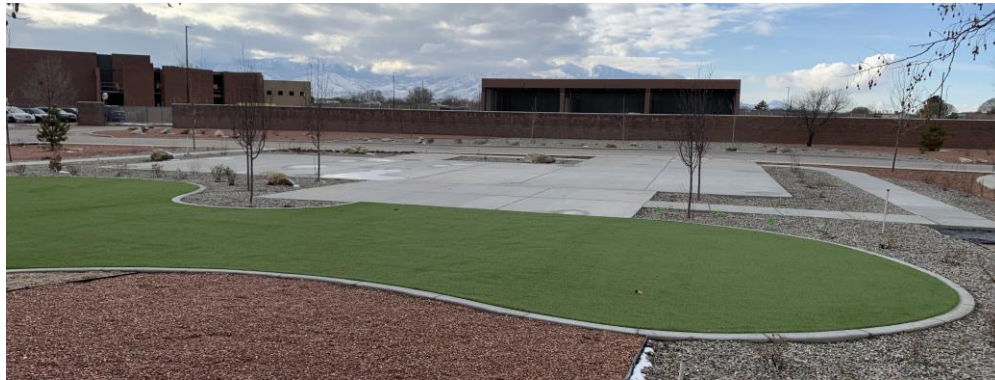
Finished concrete pad for demonstration garden area
