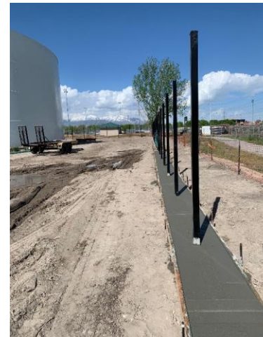
Installation of powder coated fencing along west side of property
