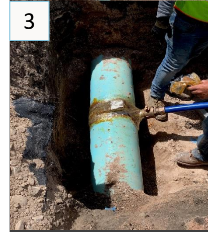
Applying wax tape and poly-ply wrap to 12"x2" brass saddle
