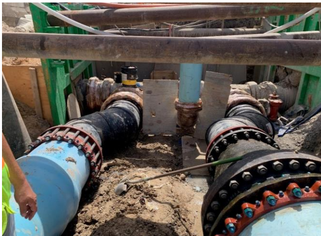
24-inch raw water and 36-inch treated water offsets
