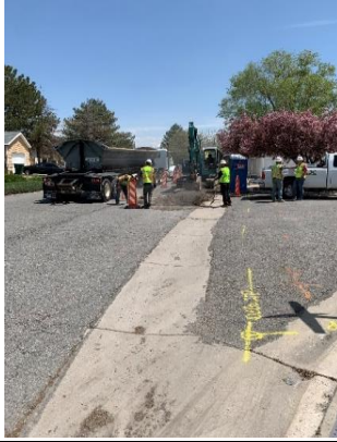
Merry Lane tie in work
