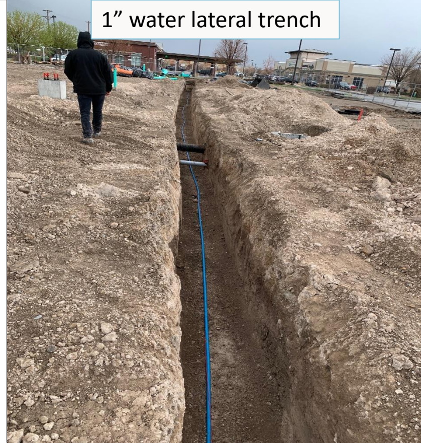
Compression fitting and tracer wire on water lateral
