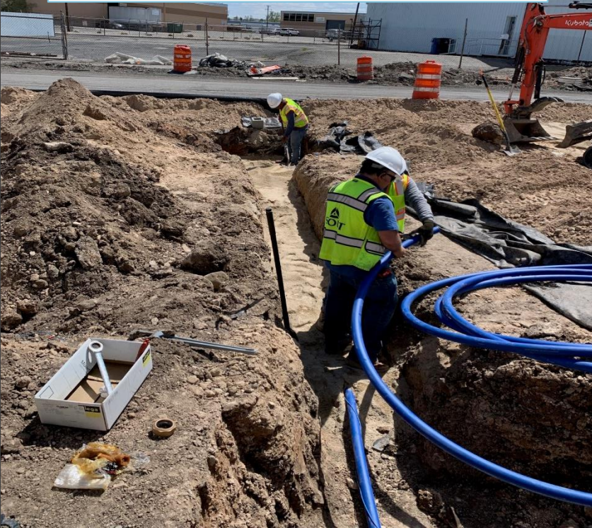
2" water lateral for landscape meter bedded in sand
