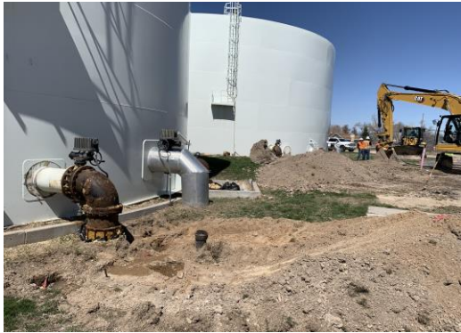
Utility potholing near 1 MG tank
