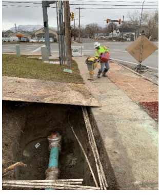
Valve repair off of Parkway Blvd
