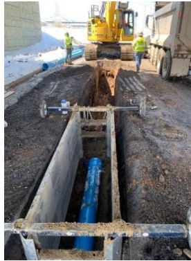
12-inch PVC installation along 4700 South
