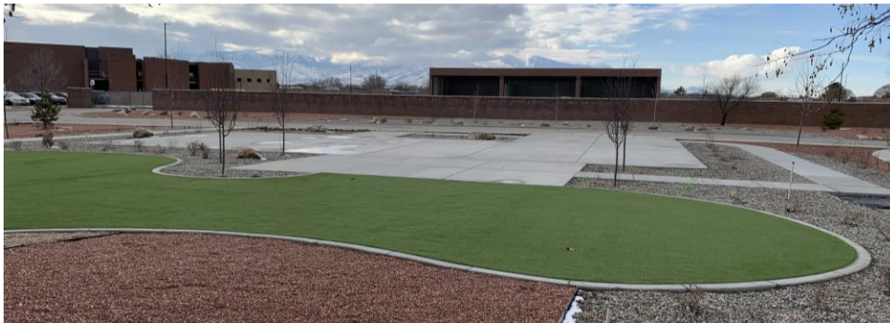
Finished concrete pad for demonstration garden area
