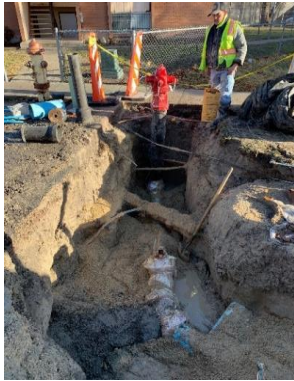
Fire hydrant installation
