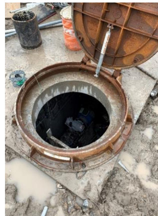
Water vault installation
