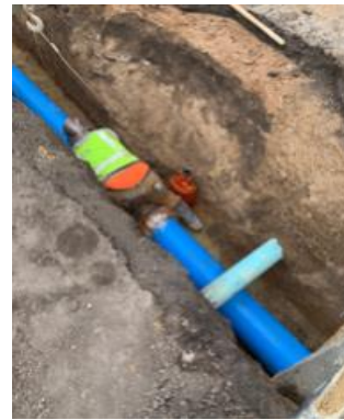
Fire Line Tee and Valve Installation
