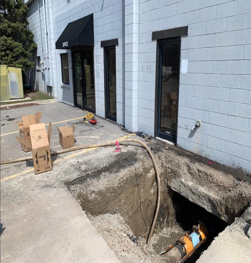
8" cast iron fire line repair
