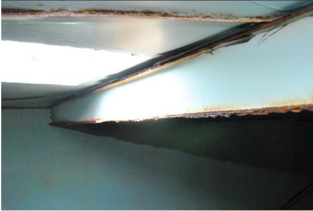
Photos of Acord Reservoir Roof Rafters Showing Extensive Corrosion
