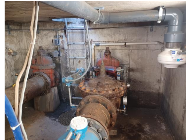
Existing Condition of Vault
