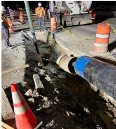
10/4/24 @ 10:42 PM: Started Pulling 24" HDPE Casing Pipe
