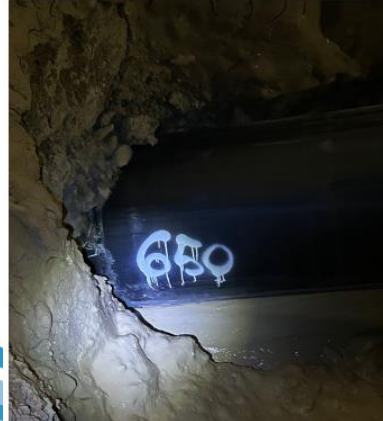
10/5/24 @ 12:53 AM: Pulled 650 LF of 24" HDPE Casing Pipe
