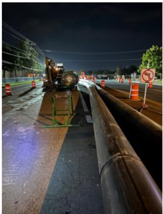
Fused 24" HDPE Casing Pipe
