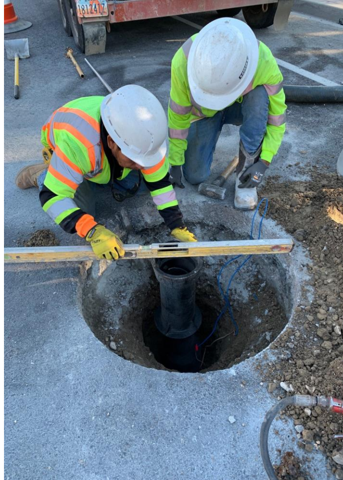
Preparing to install water valve box collar
