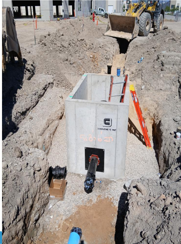
DCDA vault install
