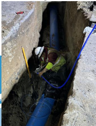
161 Service line installation
