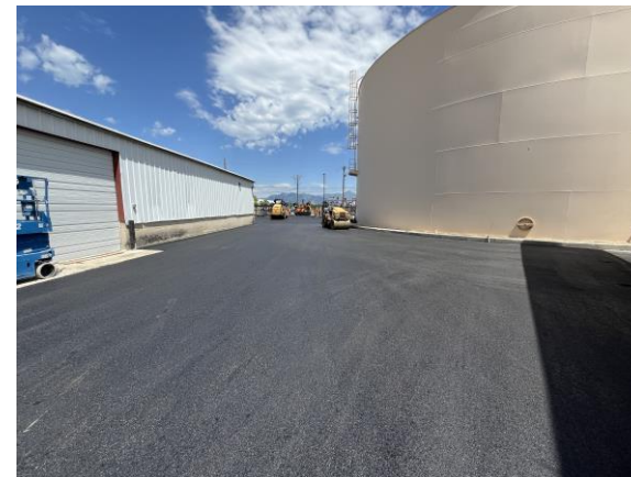
Asphalt Site Paving
