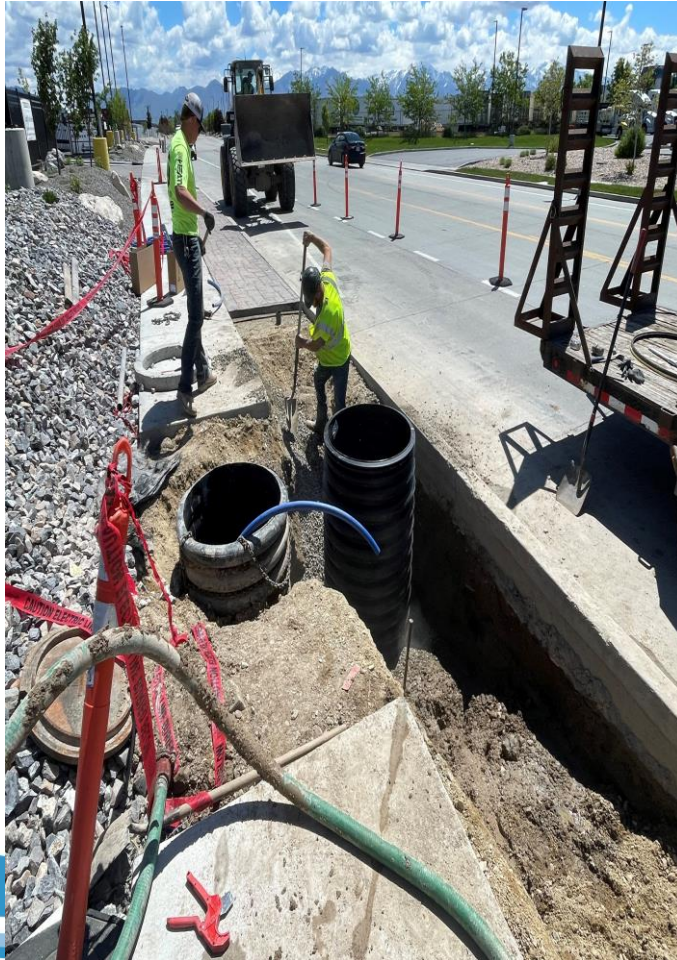
Meter being moved from future sidewalk
