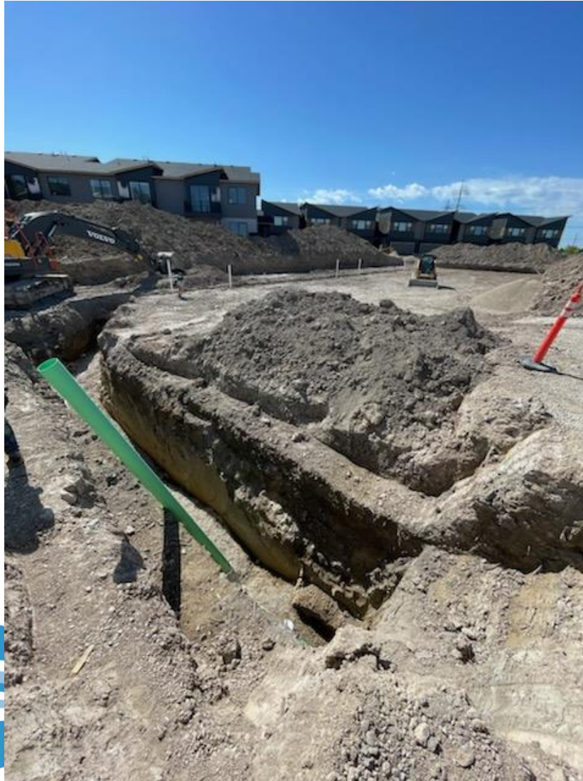
Building 18 sewer lateral inspection
