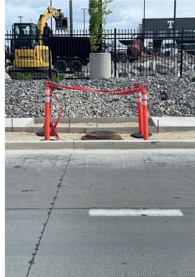
Meter relocated into park strip
