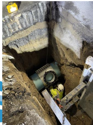
24-inch hot tap installation
