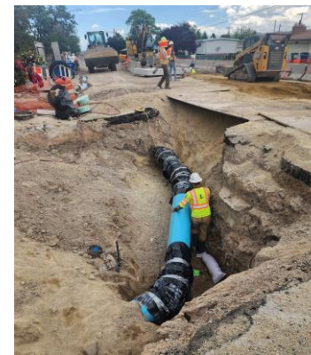
16-inch Zone 3 waterline connected to water main in 4800 West
