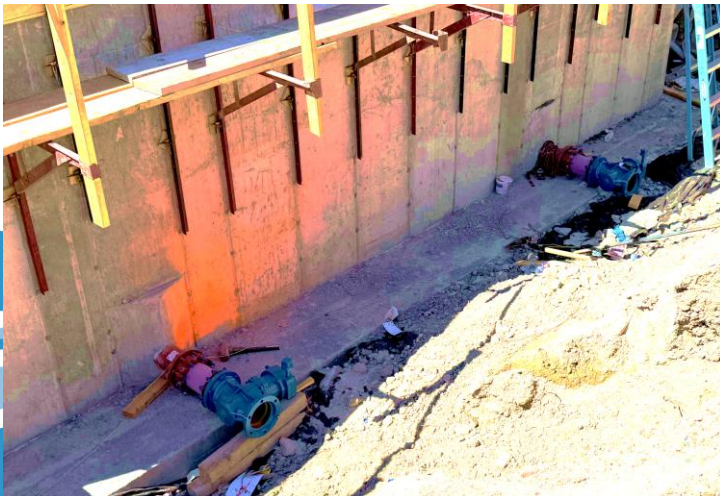
Anderson WTP Backwash Basin Roof Install and Outlet Valves
