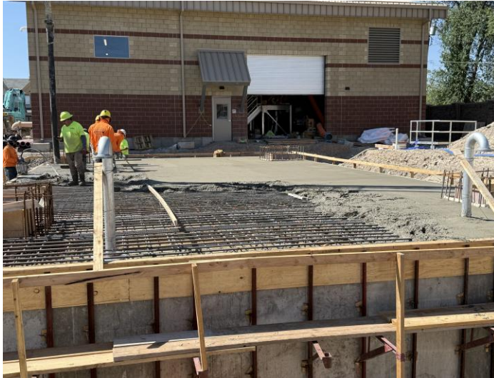
Anderson WTP Backwash Basin Roof Install and Outlet Valves
