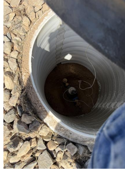
5400 West Waterline – water service and meter box install
