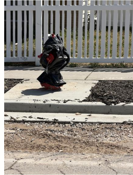
5400 West Waterline – new fire hydrants with concrete pads and SnakePits
