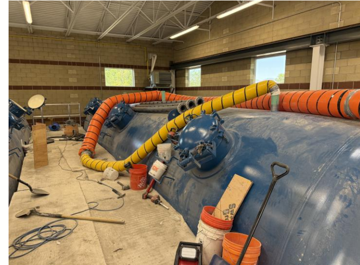
Anderson WTP Filter Vessel Internal Component Install and Internal Underdrain System
