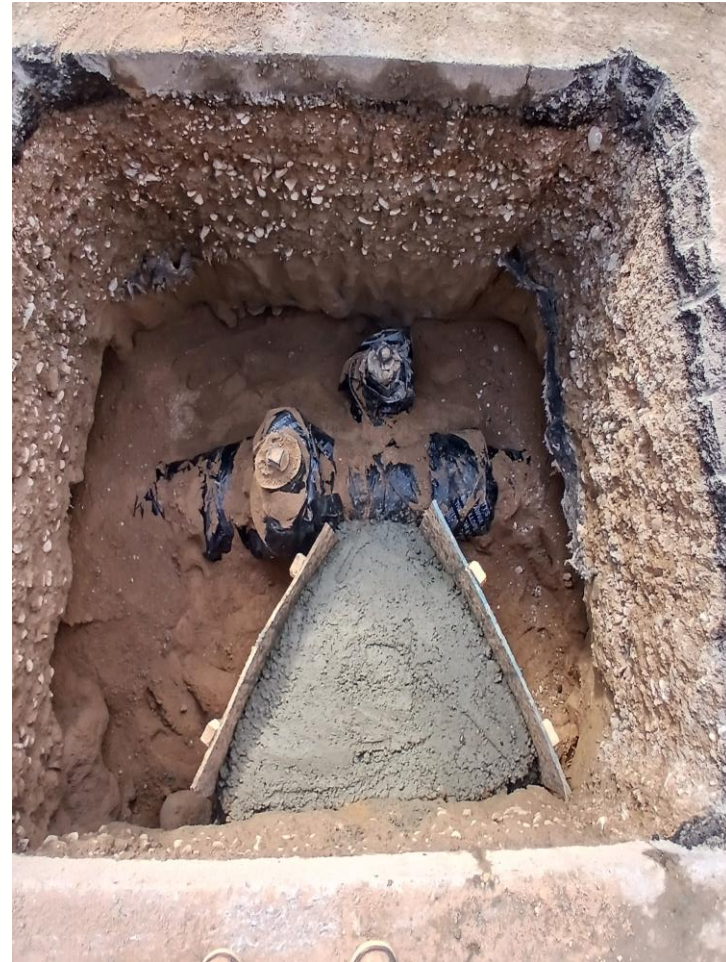
Thrust block behind 12"x6" tee
