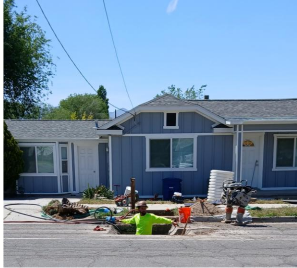
5400 West Waterline – water service and meter box install
