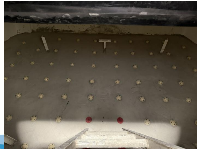
Anderson WTP Filter Vessel Internal Component Install and Internal Underdrain System
