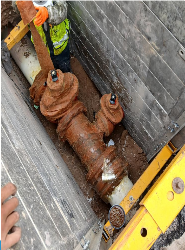
12"x6" tee and valves wax wrapped
