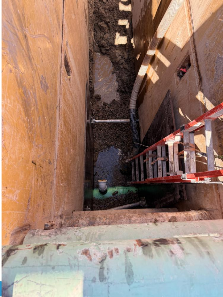
6" sewer lateral inserta tee
