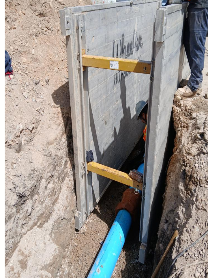
8" water line tie-in
