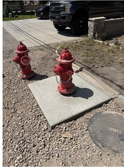
5400 West Waterline – new fire hydrants with concrete pads and SnakePits
