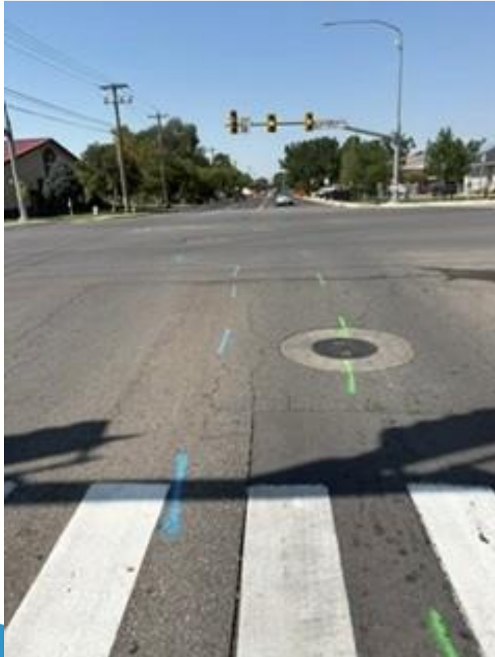
Water and sewer main blue stakes
