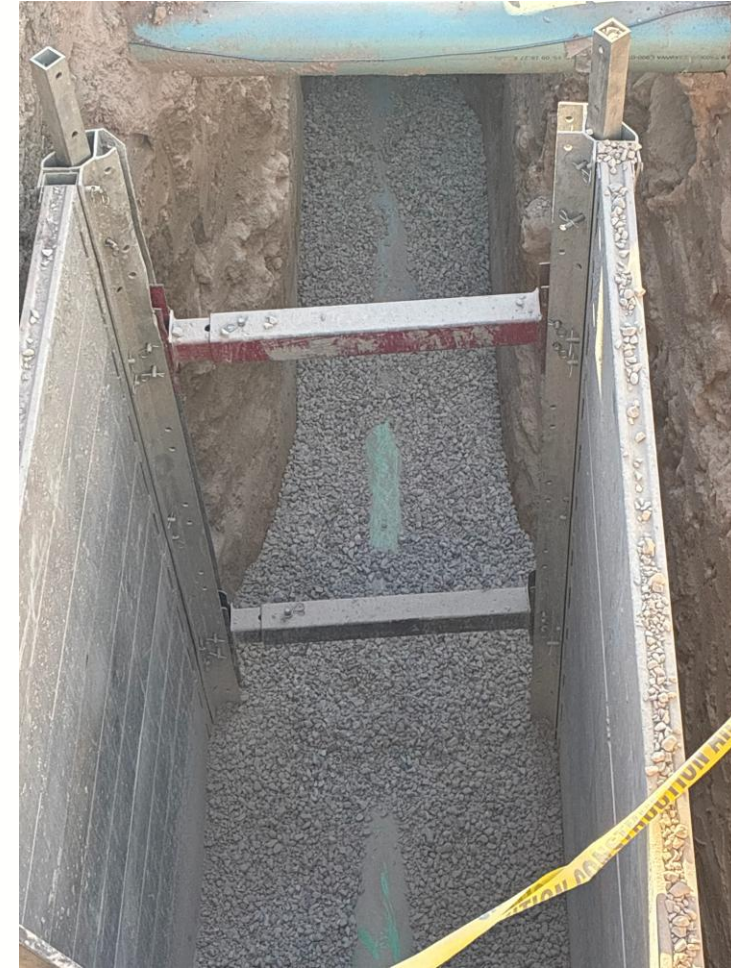
8" sewer main bedded in gravel
