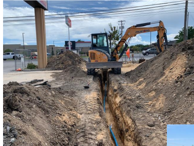
Upstream and downstream views of water lateral in trench
