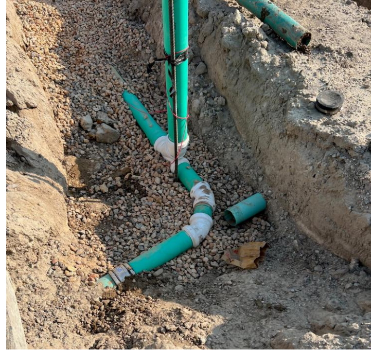
Shear band connection to existing 4" sewer
