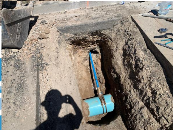
Installation of 1 ½” water service
