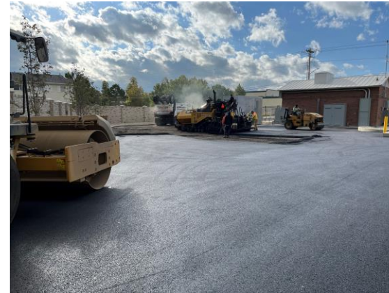
Asphalt Placement
