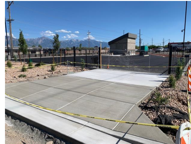
Concrete driveway entrance and asphalt pavement on site
