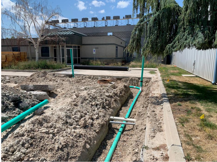
Sewer lateral cleanouts and gravel bedding
