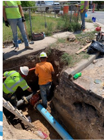
New 8" to existing 6" Connection @ King Valley Way
