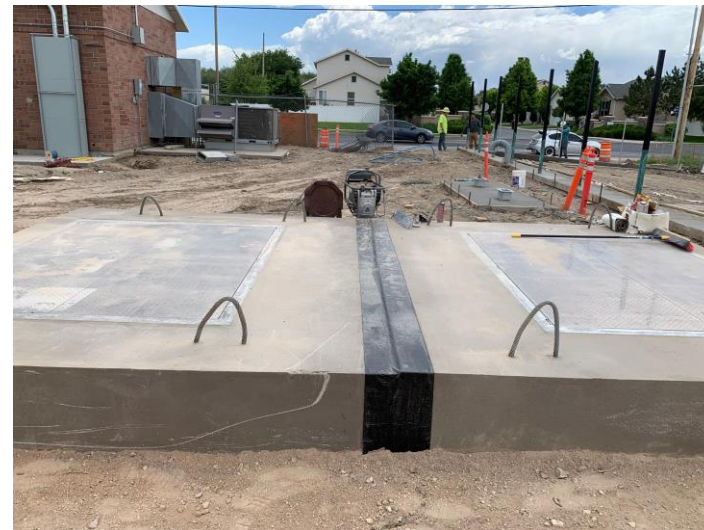
Mastic Seal Tape on Interceptor Vault
