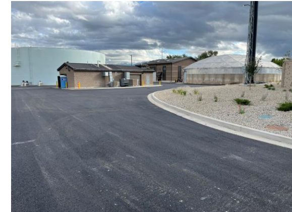
Parking Lot and Landscaping
