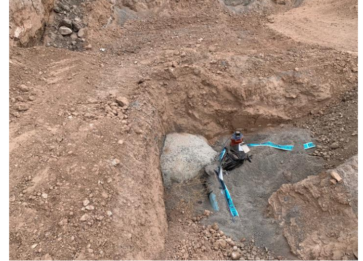
Thrust blocking on 8" waterline
