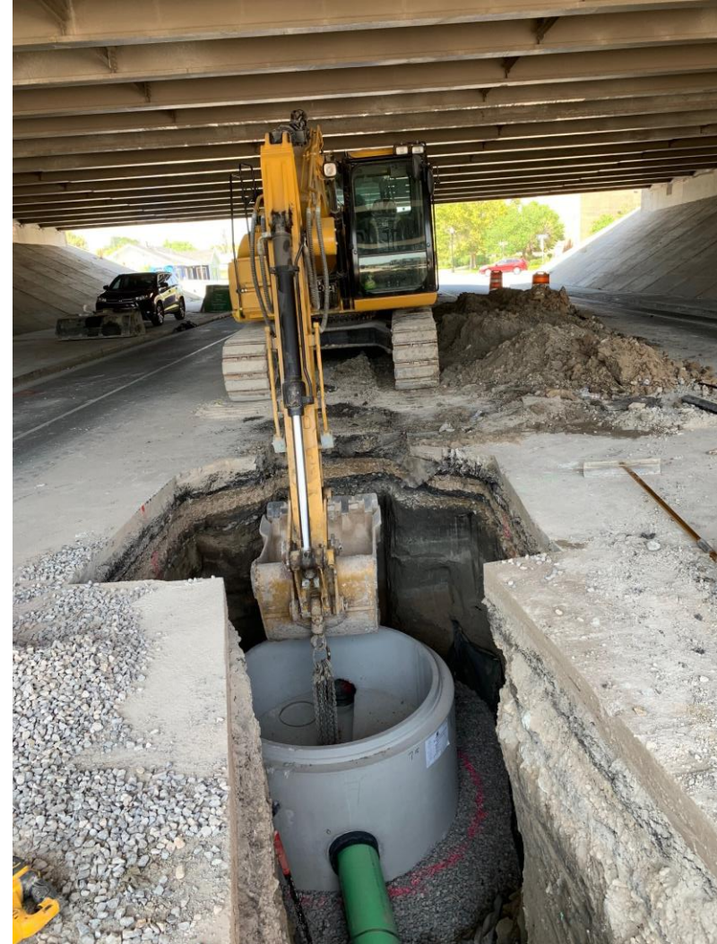
Installing sewer manhole base
