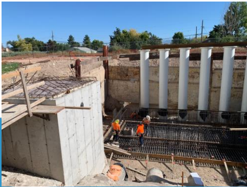
Pump station foundation rebar
