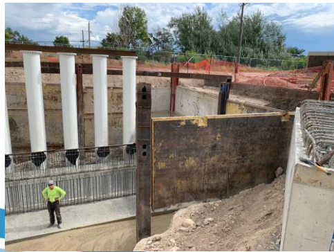
Pump station foundation concrete pad
