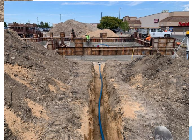
Upstream and downstream views of water lateral in trench
