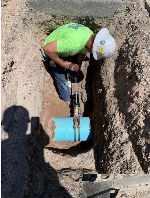
Installation of 1 ½” water service
