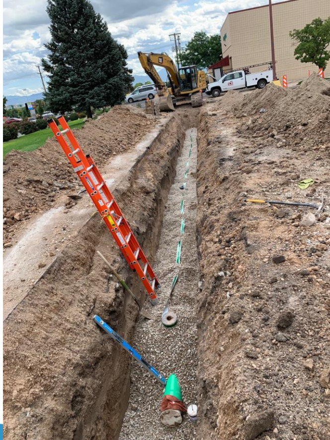
8" sewer lateral on north end of property
