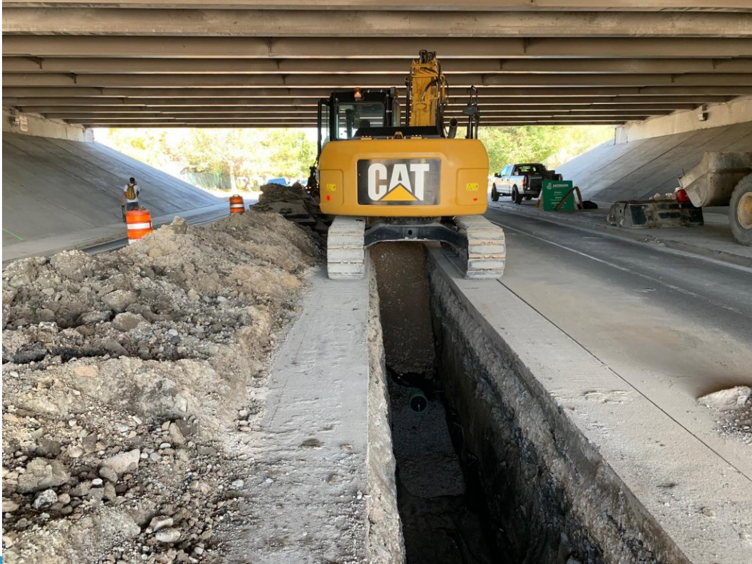
Sewer trench along 3800 S and under I-215 overpass
